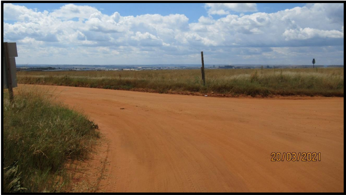
Figure 10: Existing dirt road towards newly constructed hospital.
