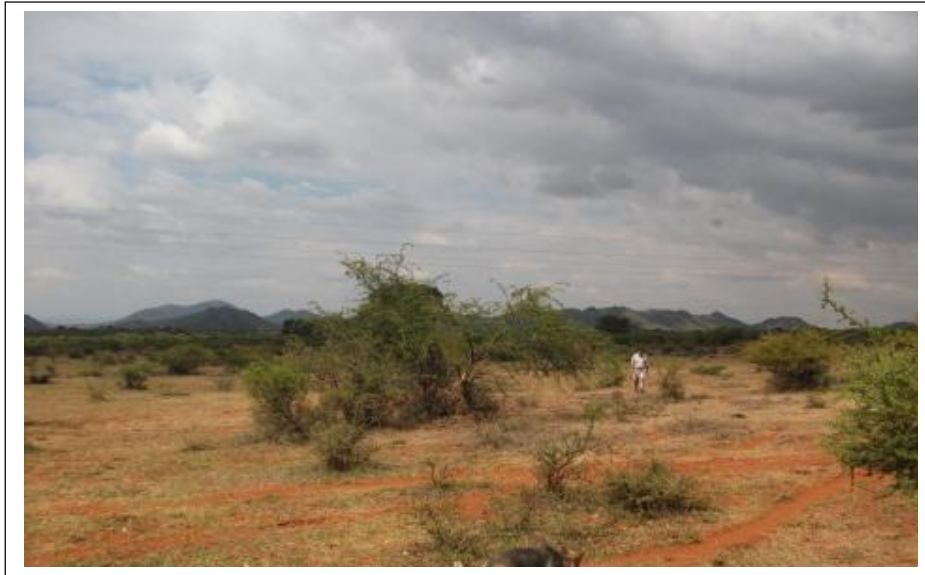
Figure 14- The proposed 132kV loop-in loop-out power line running from the Middelpunt-Dithabaneng power line to the proposed new Boynton Substation runs across abandoned agricultural fields on the farm Mphatlele 457KS.
