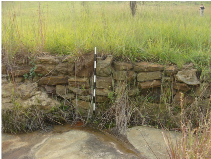
Figure 20 Possible dam wall at site no. 13.
