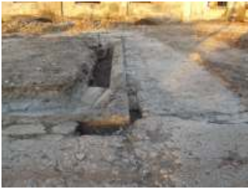
Figure 12: NE corner of cooling pond exposed.
