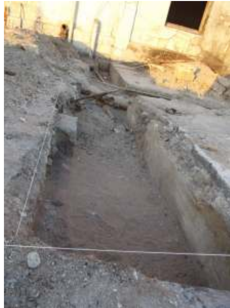
Figure 10: Pipes in the east wall of cooling Pond (trench 2).
