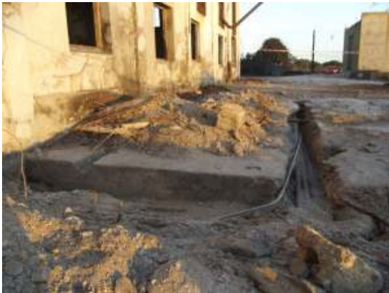
Figure 9: View of the gravity tank and pipes in front of power station.
