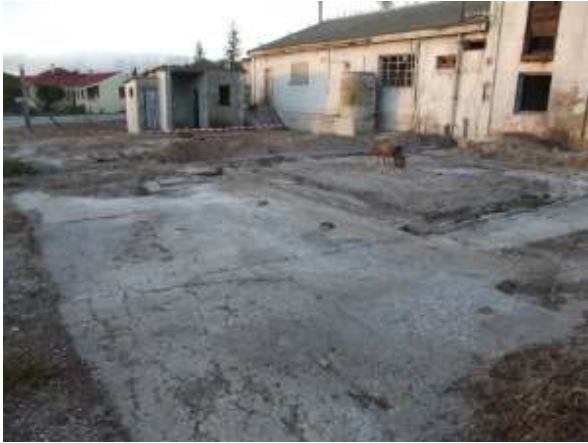
Figure 6: View of cement capping in front of Power Station.
