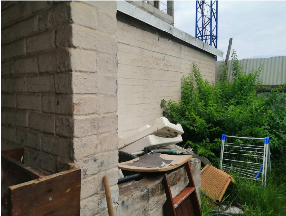
existing house on site-rear view
