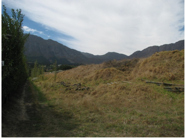
VIEW OF THE DAM WALL
