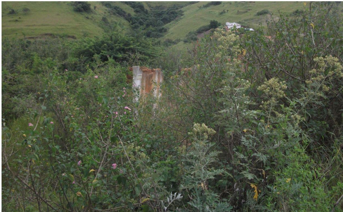
Figure 15: Remains of white painted structure
