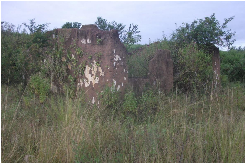
Figure 6: Partly demolished dwelling
