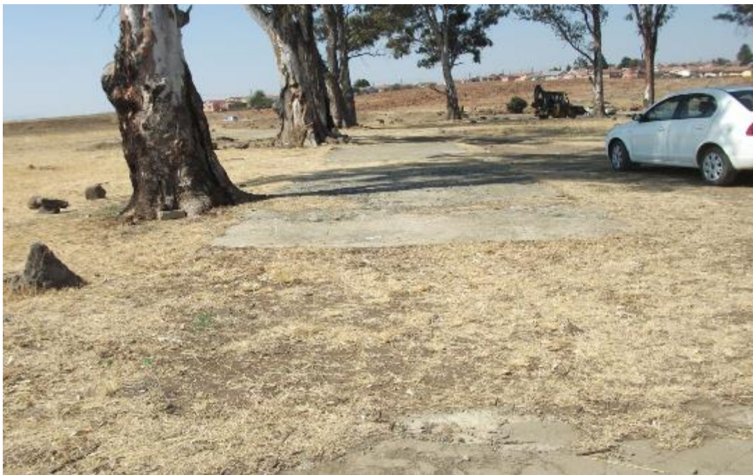
Figure 8: Remains of structure/s
