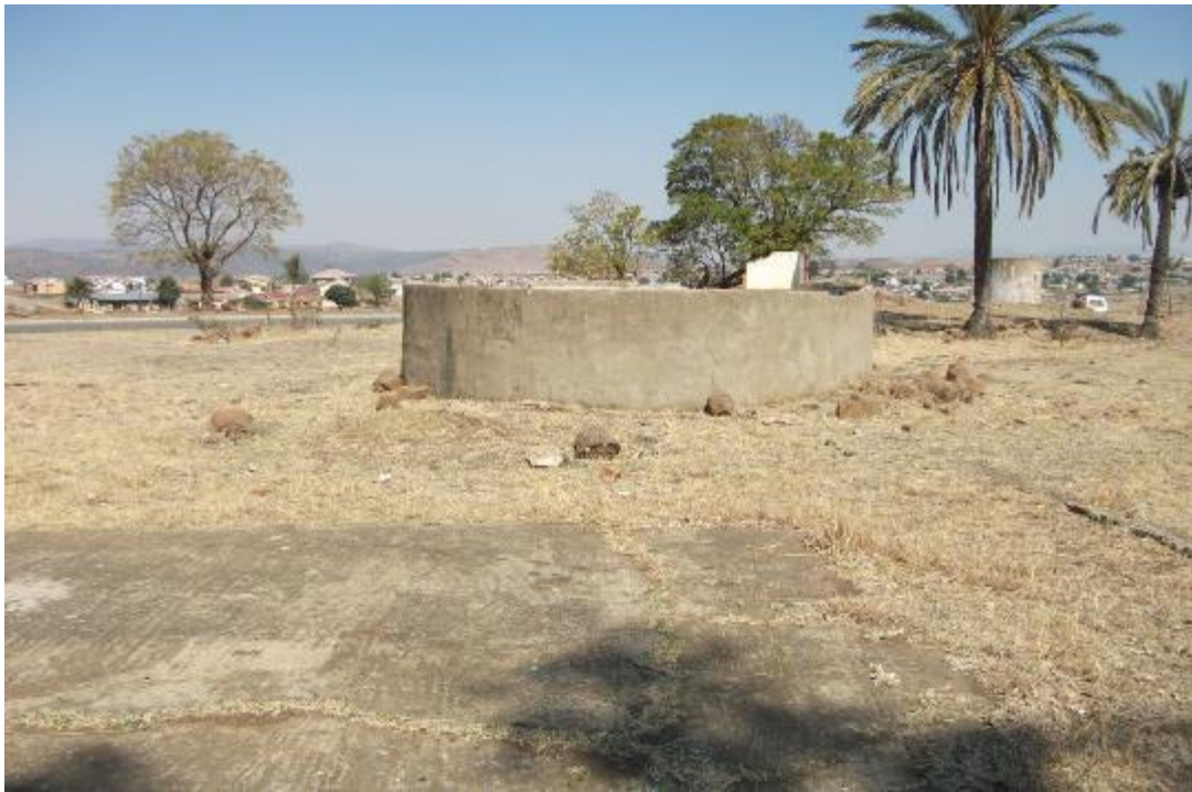
Figure 9: Floor of structure, reservoir and other remains
