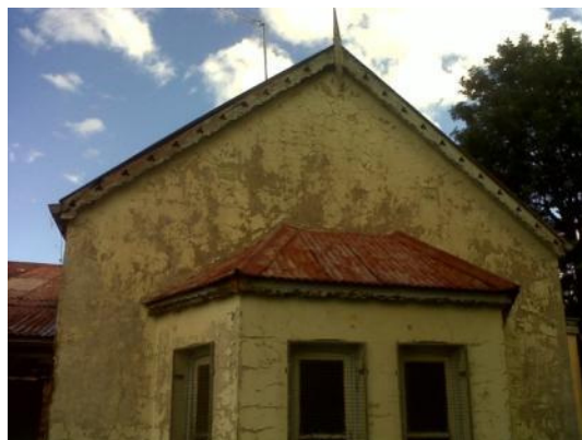
Fig 20: Front bay, north elevation
