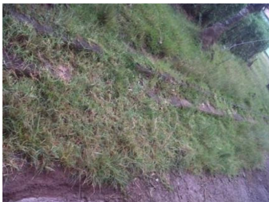
Fig 26: Water furrow along access road
