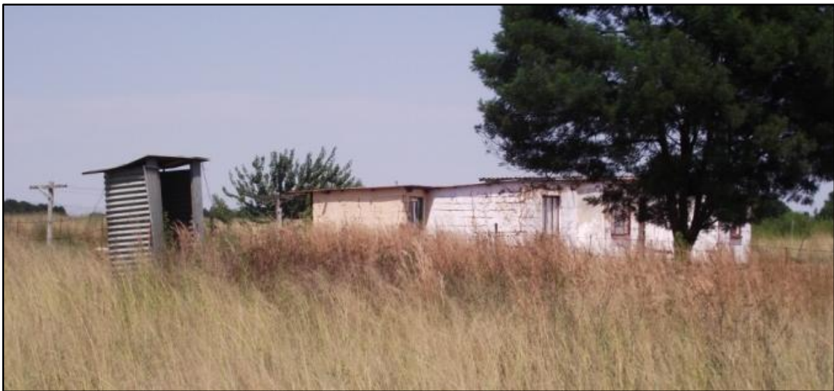
Figure 9 – MF 001, View of worker houses (MF 001/3)
