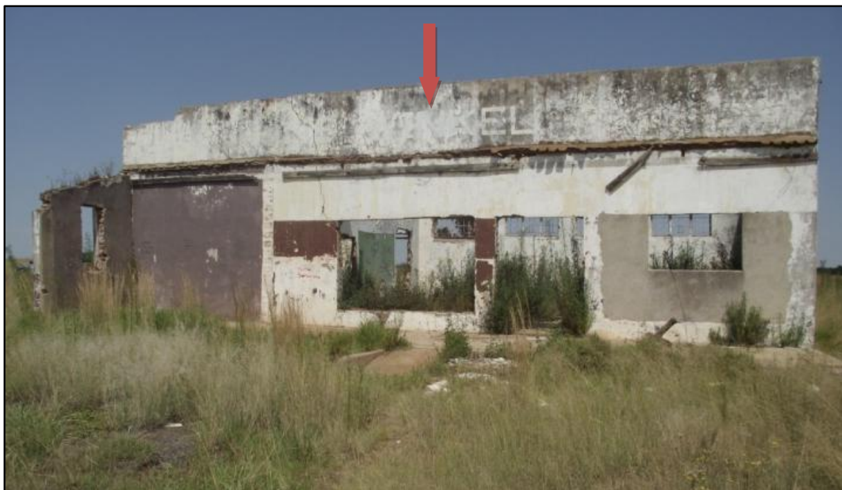
Figure 12 – MF 002, Shop building – front (arrow indicates faded remains of sign - “winkel”)
