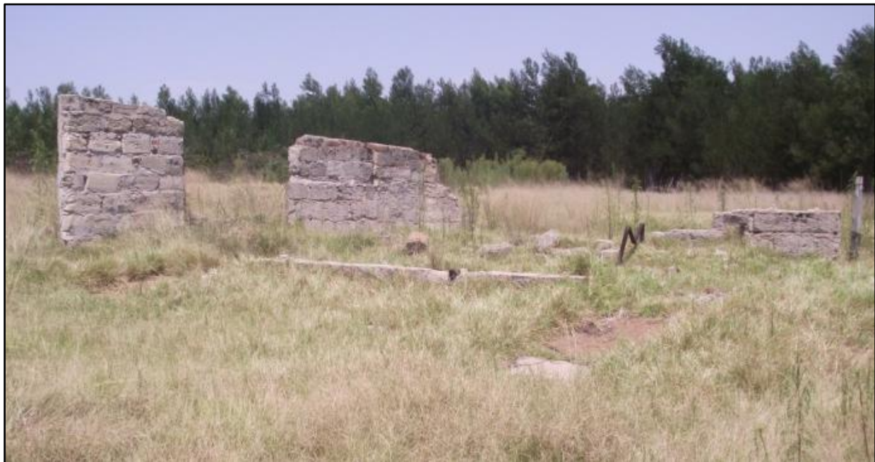
Figure 18 – MF 003, Cement-brick outbuilding, on western side of house
