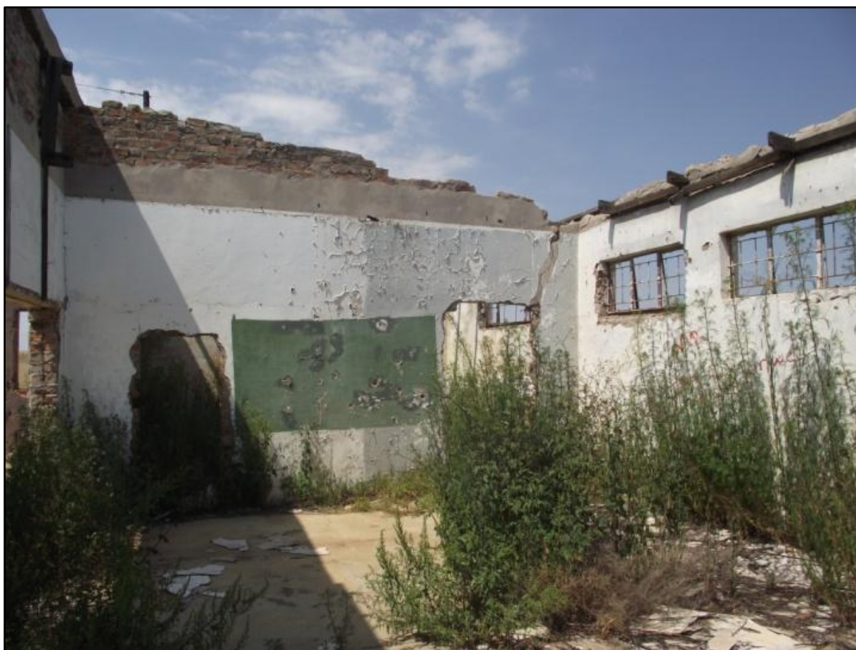
Figure 13 – MF 002, Shop building - inside
