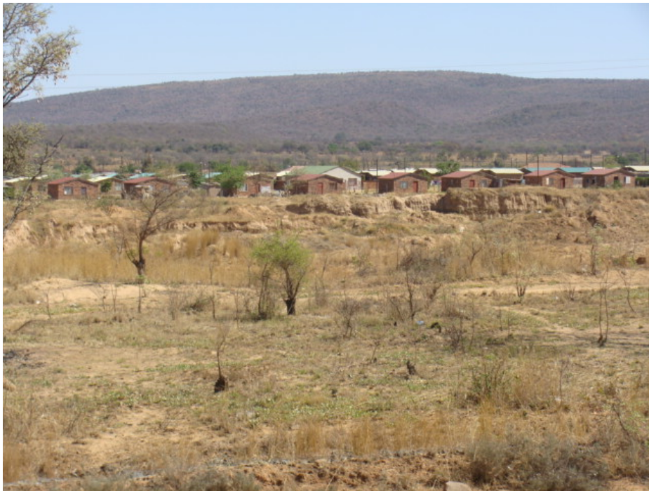
Figure 10: Houses adjacent to the surveyed area.
