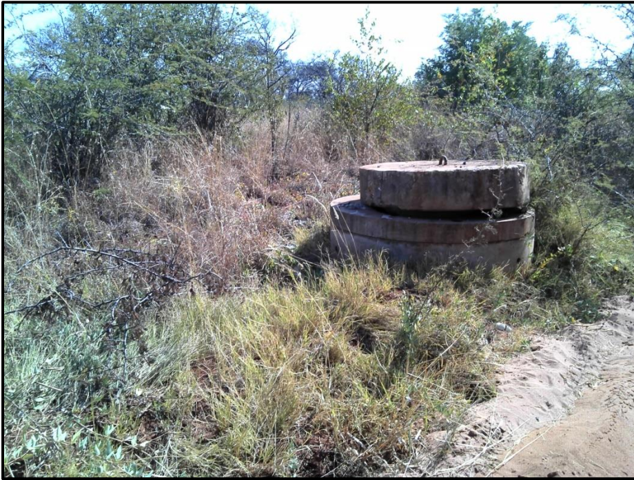
Figure 5. Existing water supply line.
