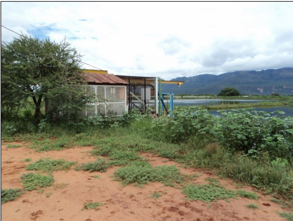
Figure 17: POI f at Oxidation Pond B.
