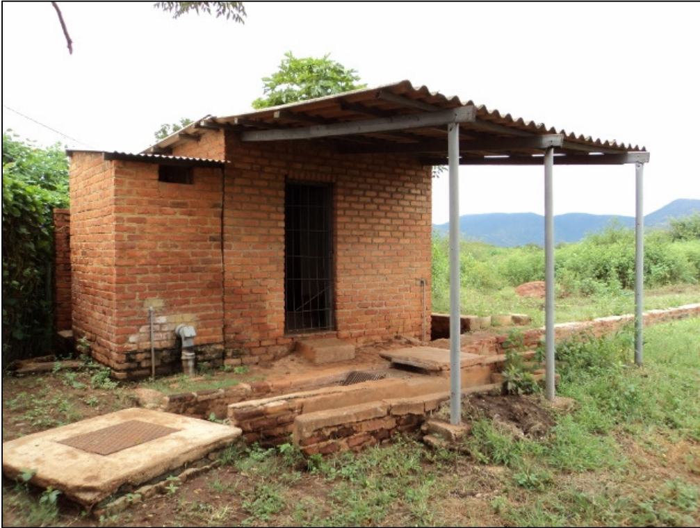
Figure 14: POI b at Oxidation Pond A.
