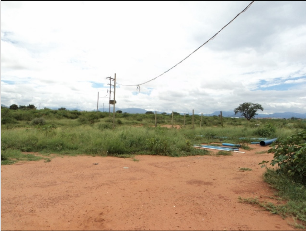
Figure 8: More accessible section at Oxidation Pond B.
