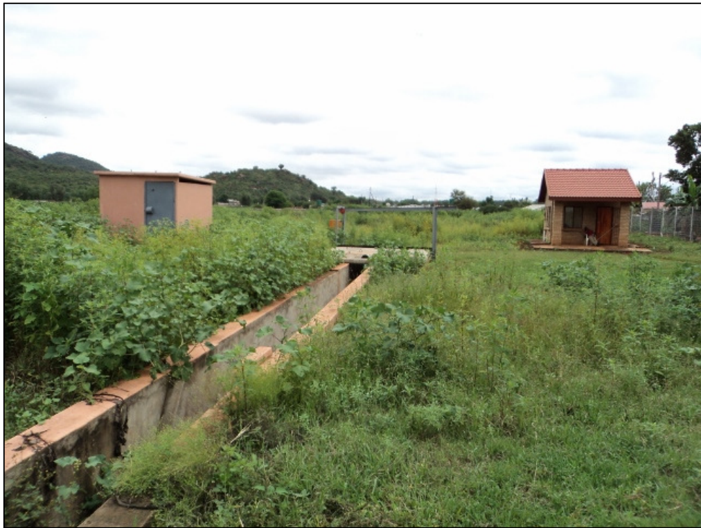
Figure 13: POI a & c at Oxidation Pond A.
