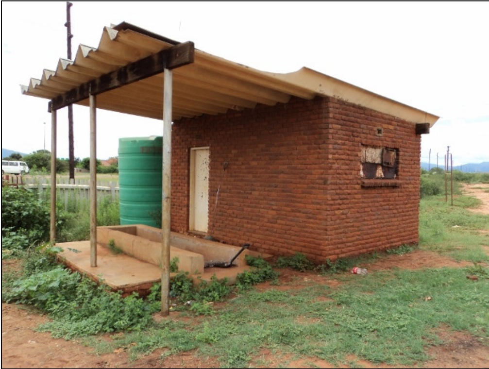
Figure 16: POI e at Oxidation Pond B.
