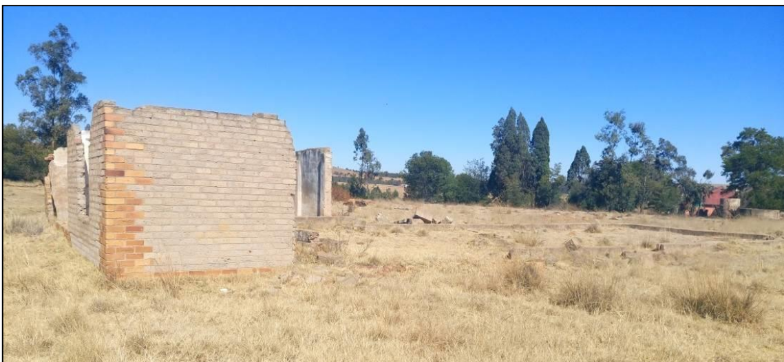
Figure 14: View of the north wall of a second outbuilding to the south of the main dairy building. Some cement foundations are visible to the right. Again, modern bricks are evident.
