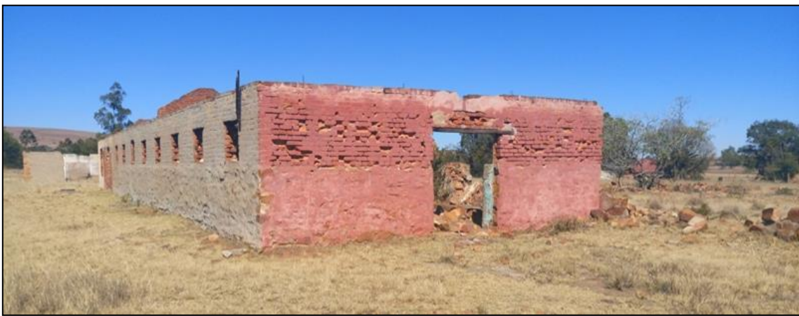
Figure 13: View of the northern wall of the main dairy building showing modern bricks with a concrete lintel above the doorway. The stone and cement kraal is visible to the right.
