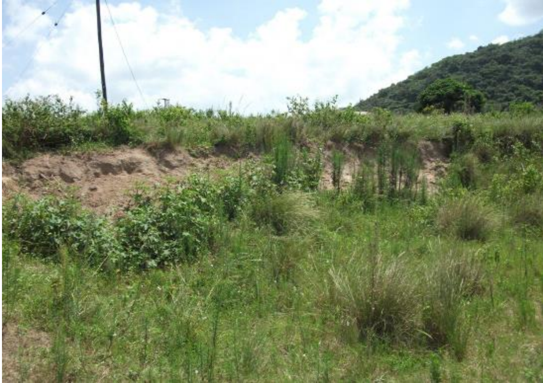
Figure 7: Soil removal and section of pylon
