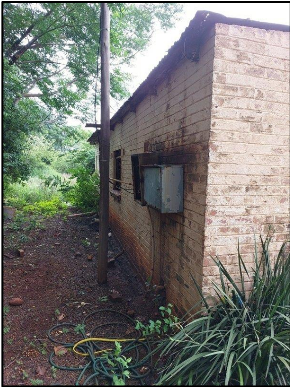
Figure 7.13. Secondary labourer's house situated along the western edge of the proposed project area south of the main house. - West facing.
