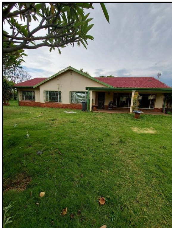
Figure 7.8. View of the main house situated on the property - North facing.
