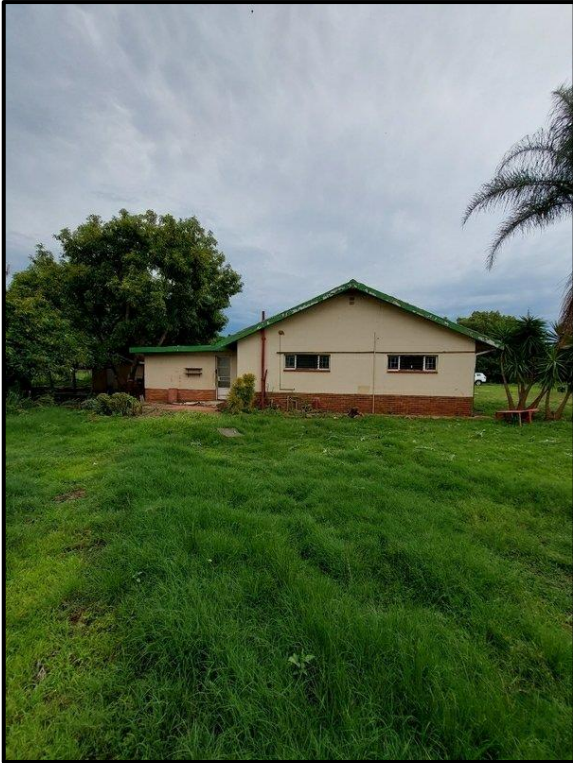
Figure 7.9. View of the main house situated on the property - East facing.
