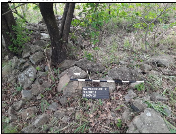
Figure 8. Northern elevation of Feature 1.
