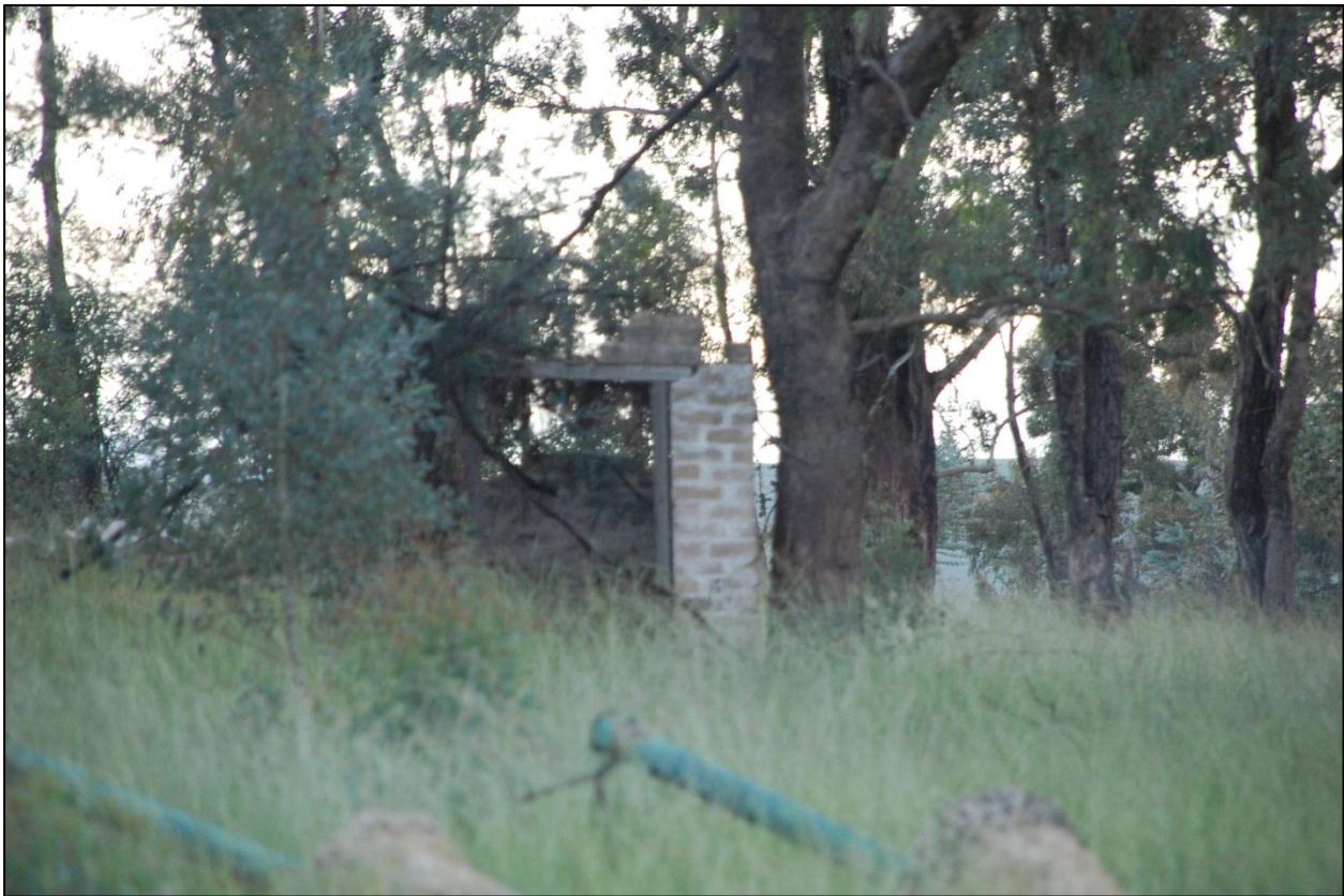
Photo 2 Dilapidated Modern Structures
