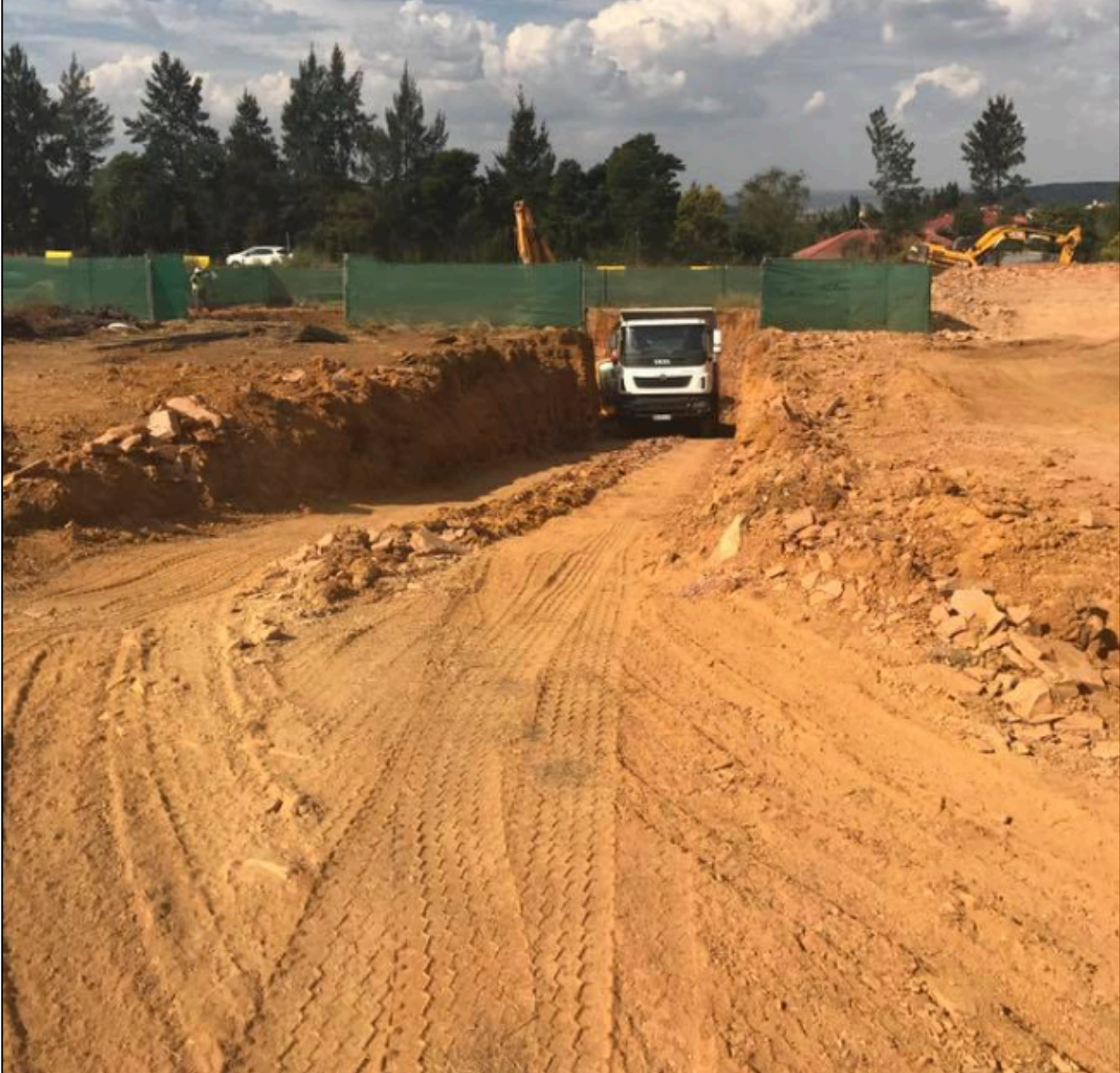
Figure 6. Eastern Border of the Study Area (heavy excavations been done)
