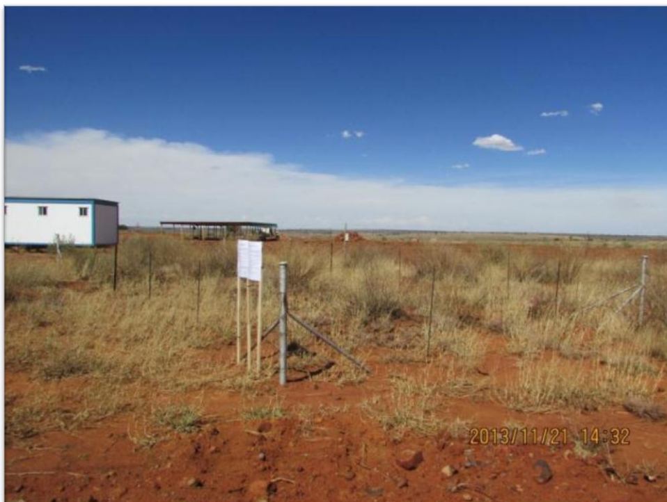
Figure 28: Site notices with construction office in background
