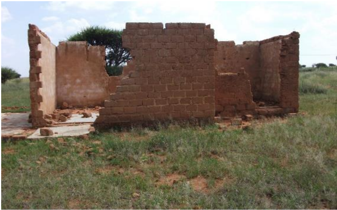
Figure 10: Remains of brick structure
