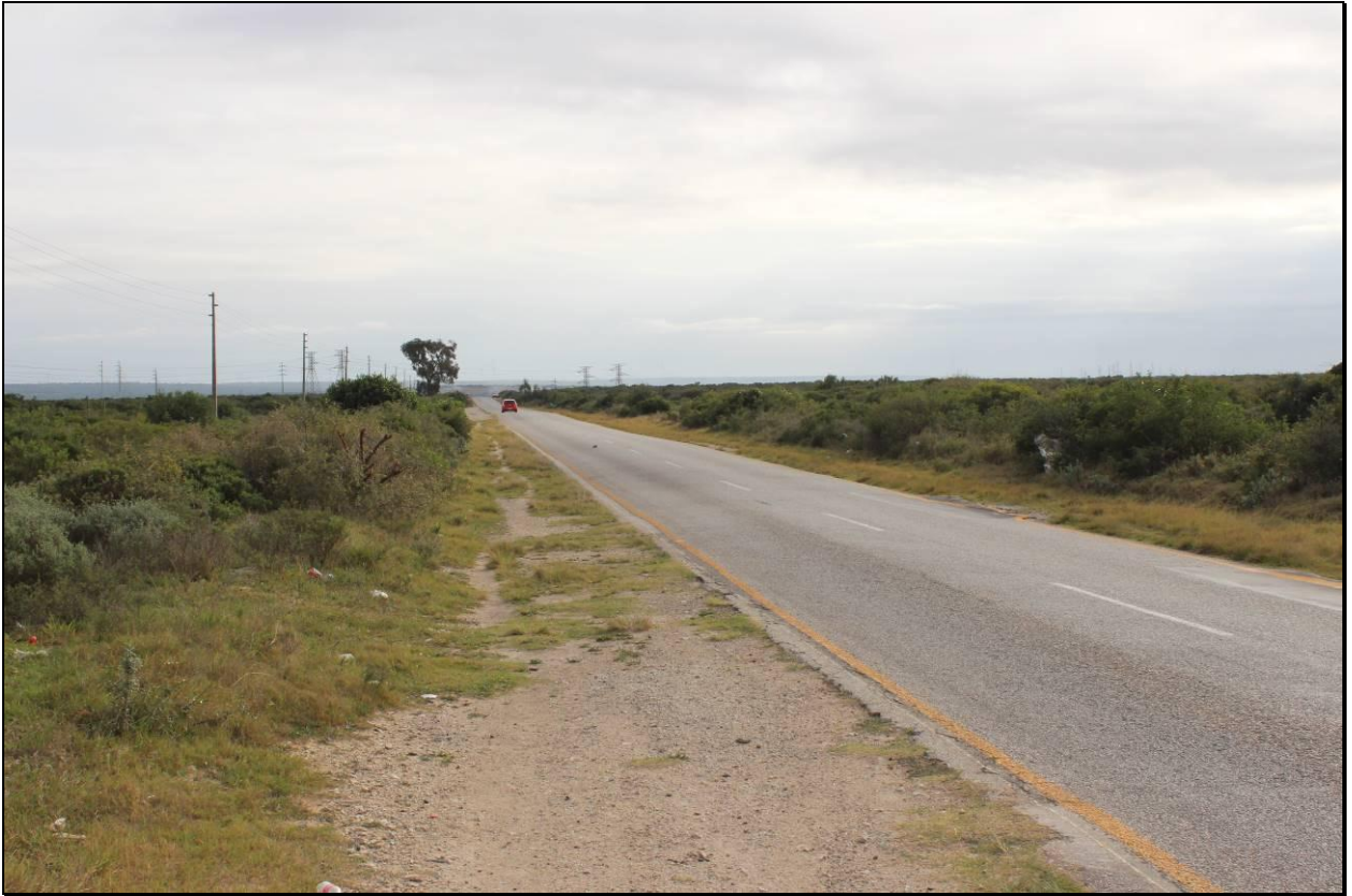
Figure 4. Beginning of the Motherwell Addo road upgrade (Algoa Group).
