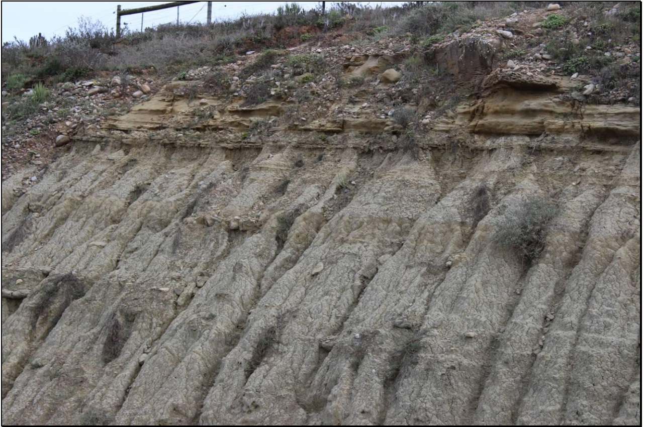
Figure 8. Sundays River Formation exposed in the road cutting near the end of the upgrade.
