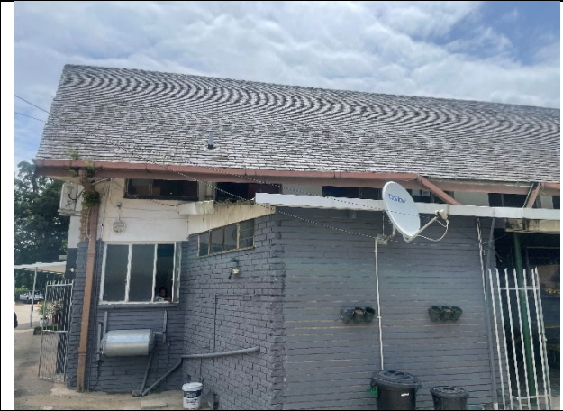
Exterior Photograph No 1 of existing Structures
