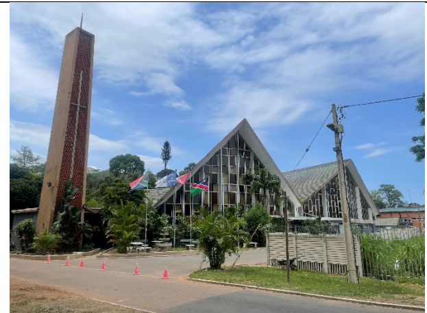
Exterior Photograph No 1 of existing Structures
