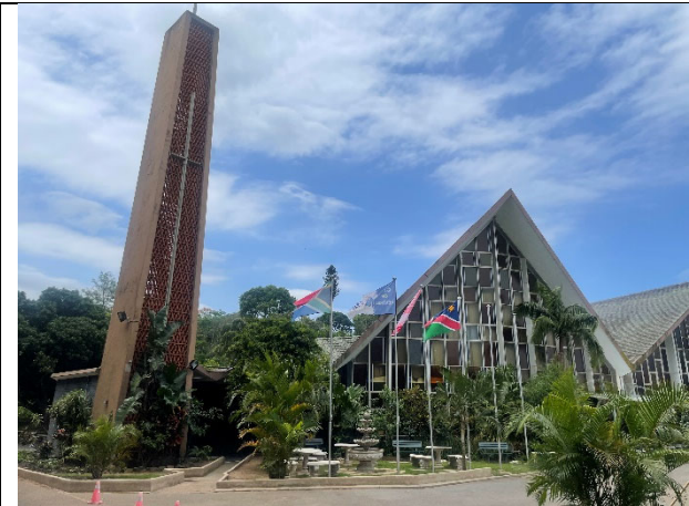
Exterior Photograph No 1 of existing Structures
