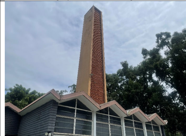
Exterior Photograph No 1 of existing Structures
