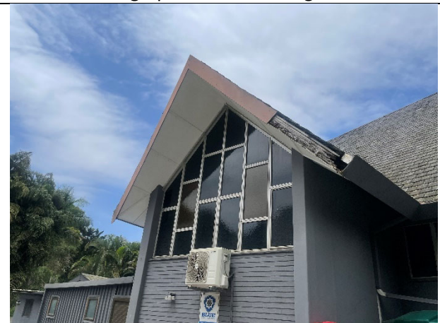
Exterior Photograph No 1 of existing Structures
