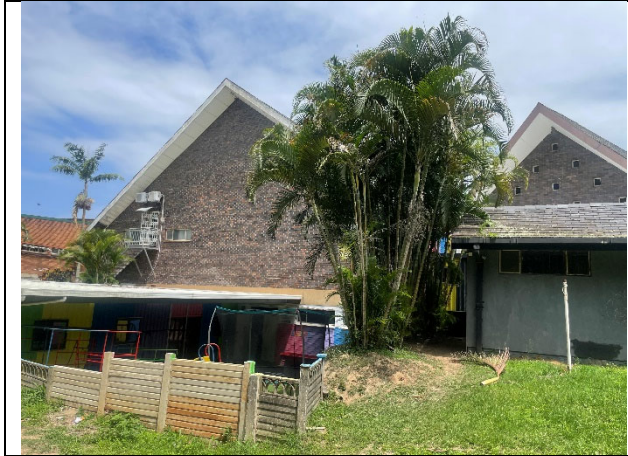
Exterior Photograph No 1 of existing Structures
