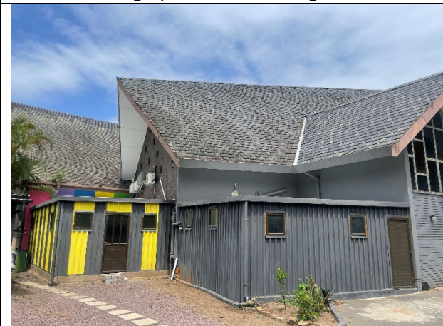
Exterior Photograph No 1 of existing Structures
