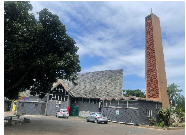
Exterior Photograph No 1 of existing Structures
