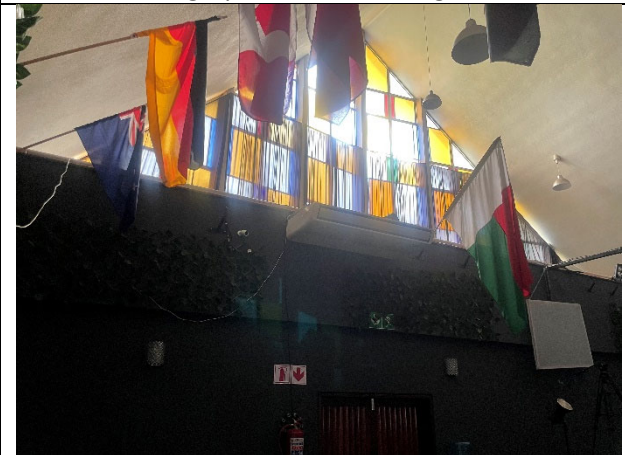
Interior Photograph No 1 of existing Structures
