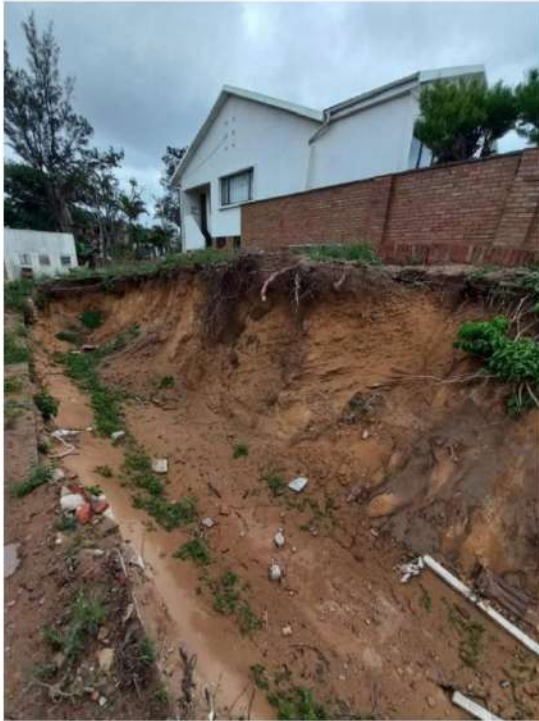
SLIDE 1 : EXCAVATED EASTERN EMBANKMENT
