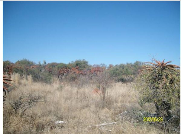
Fig 2. General view of site affected by the power cable
