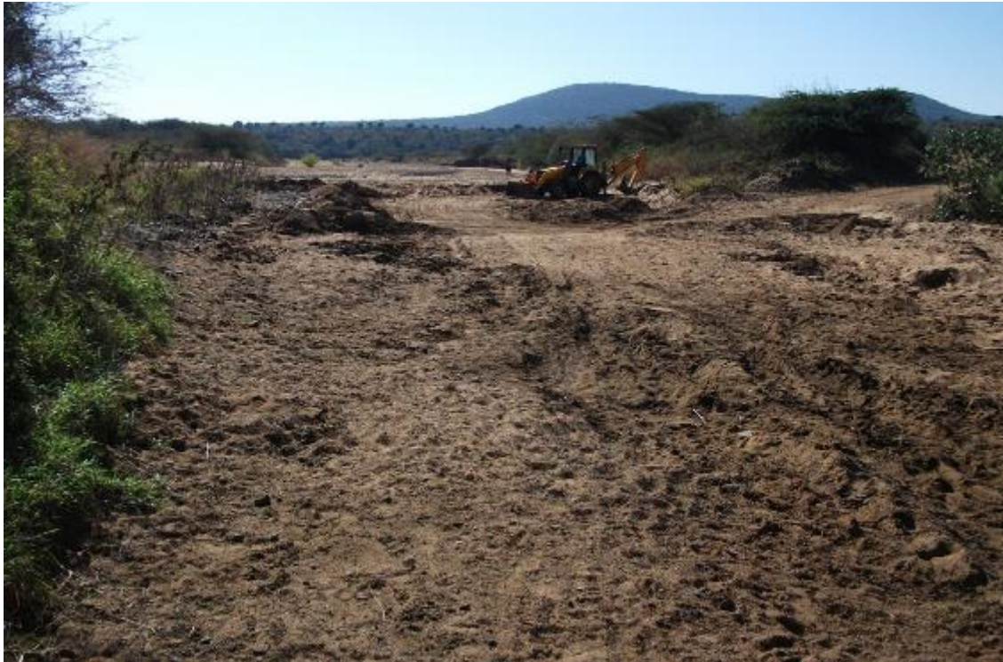
Figure 3: Dry river bed with work taking place looking northwards
