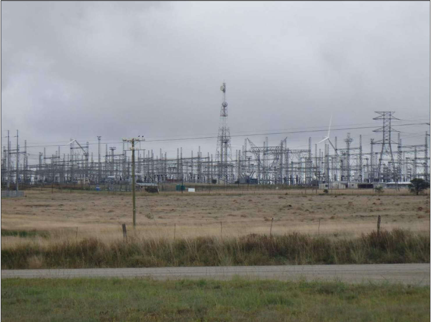
Figure 5.13: Contextual Images of Development Area indicating existing substation infrastructure
