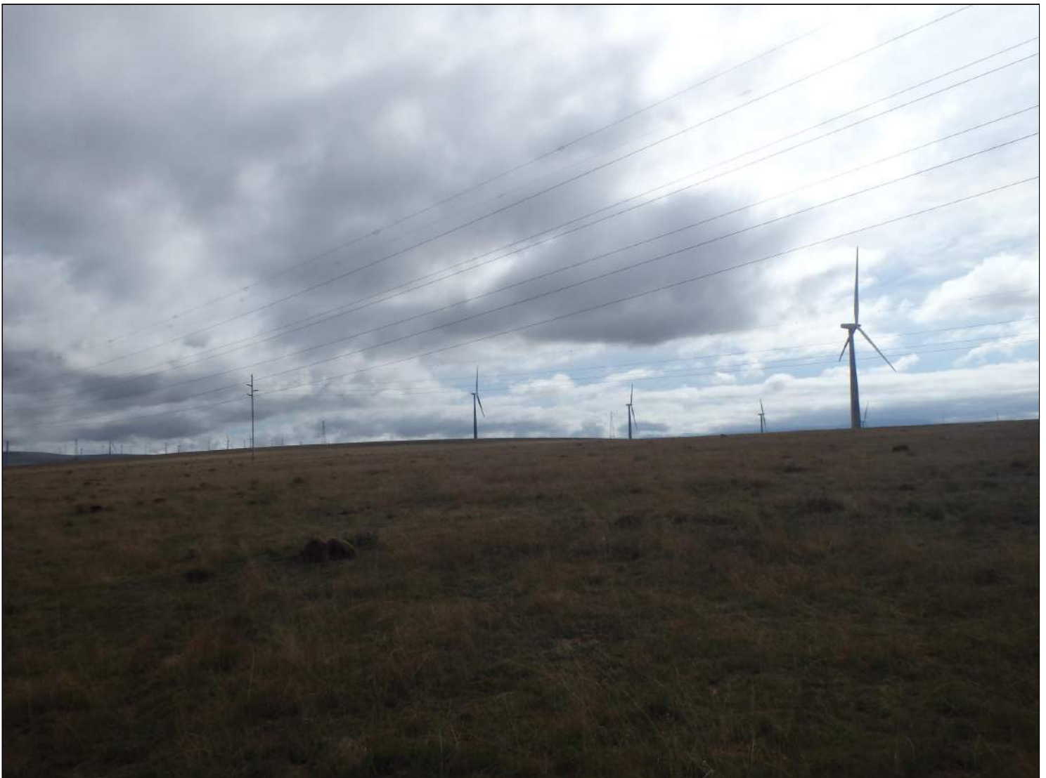
Figure 5.12: Contextual Images of Development Area indicating existing turbines and OHL infrastructure adjacent to the development area
