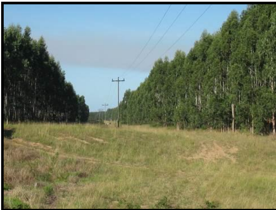
Figure 7. Much of the preferred powerline route is covered by commercial forestry plantations.
