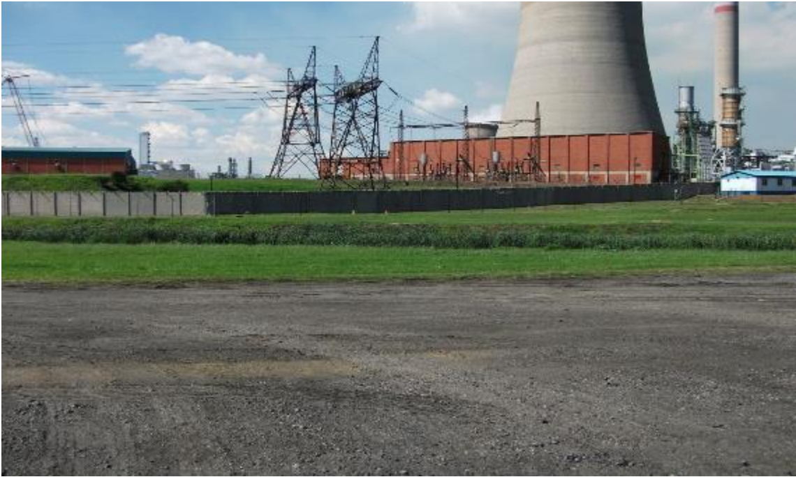
Figure 20: View of existing power lines and OCGT in background
