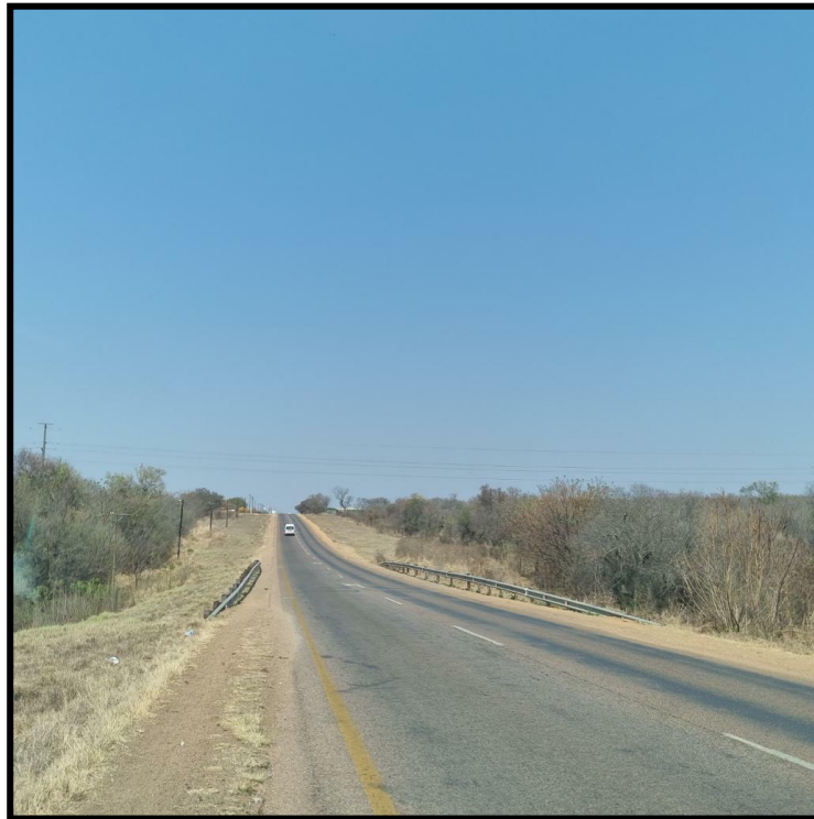
FIG. 9: CULVERTS ON THE N11
