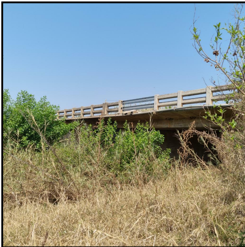
FIG. 8: MOSES RIVER BRIDGE
