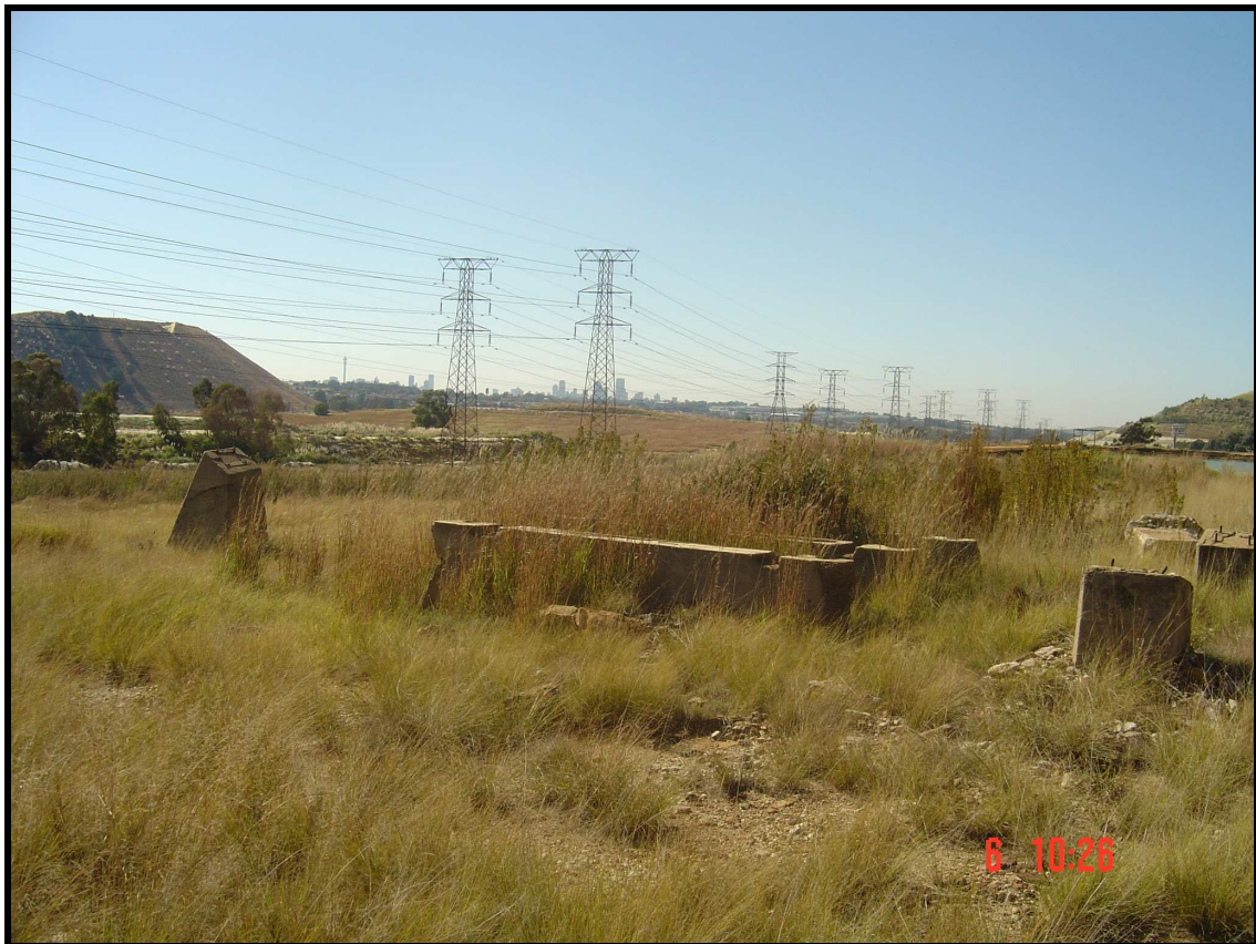
Figure 5 – Concrete pillar foundations
