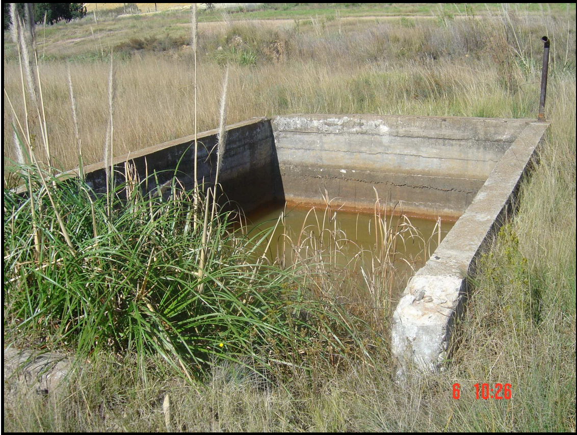
Figure 6 – Shaft collar
