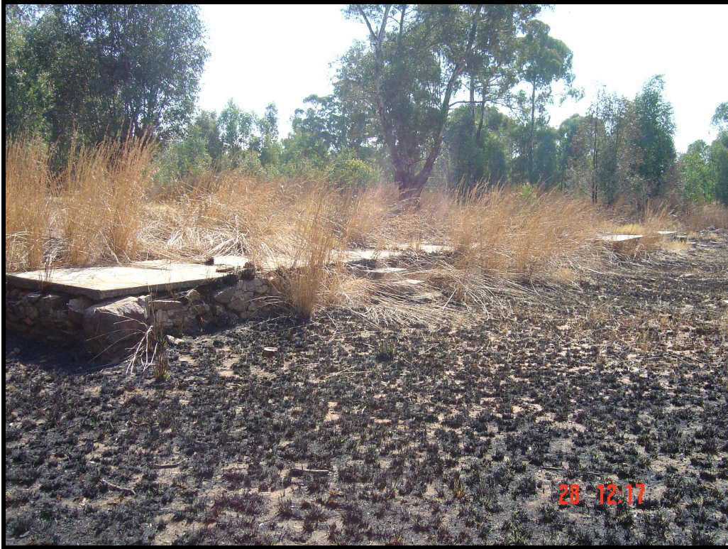
Figure 12 – Old structure foundation
