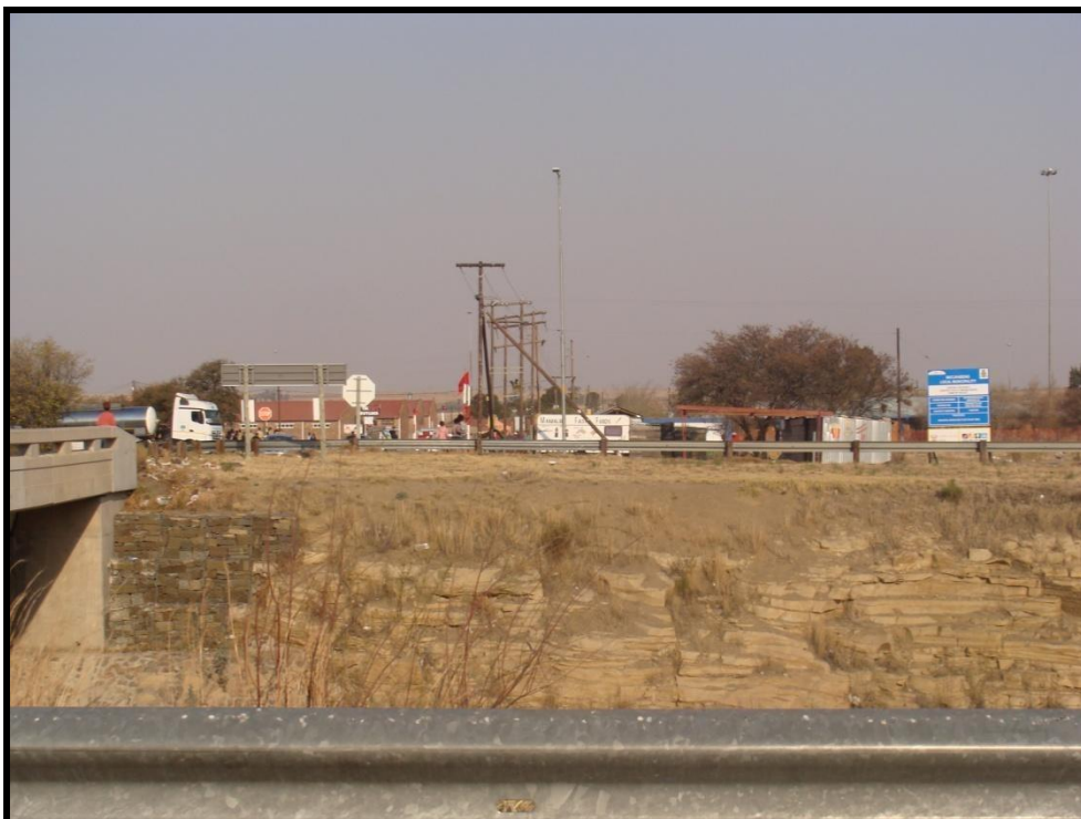
Figure 2: Photograph taken behind N1 Bloemfontein sign shown in Figure 1, showing the bridge crossing the N1 highway on the left of the image. As can be seen in the road cutting, fine-grained sandstone is exposed to the east and west of the highway
