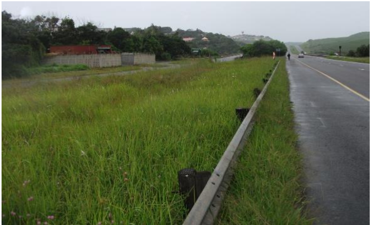
Figure 16: View of eastern embankment of N2 before Lovu River
