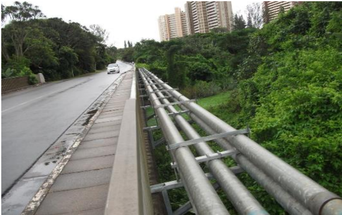
Figure 13: R102 road crossing Little Manzimtoti River with pipelines attached to it
