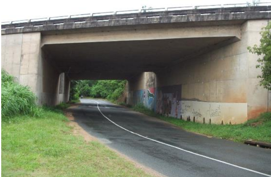
Figure 15: Underpass in Warner Beach
