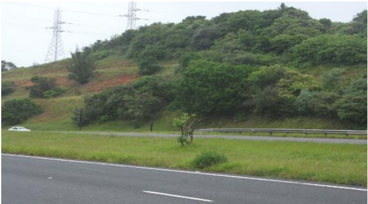
Figure 12: Steep terraced embankments with power lines in background
