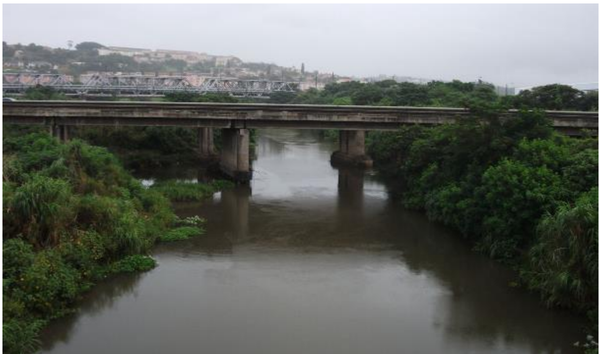
Figure 5: View of Mbokodweni Bridge with Railway Bridge in background
