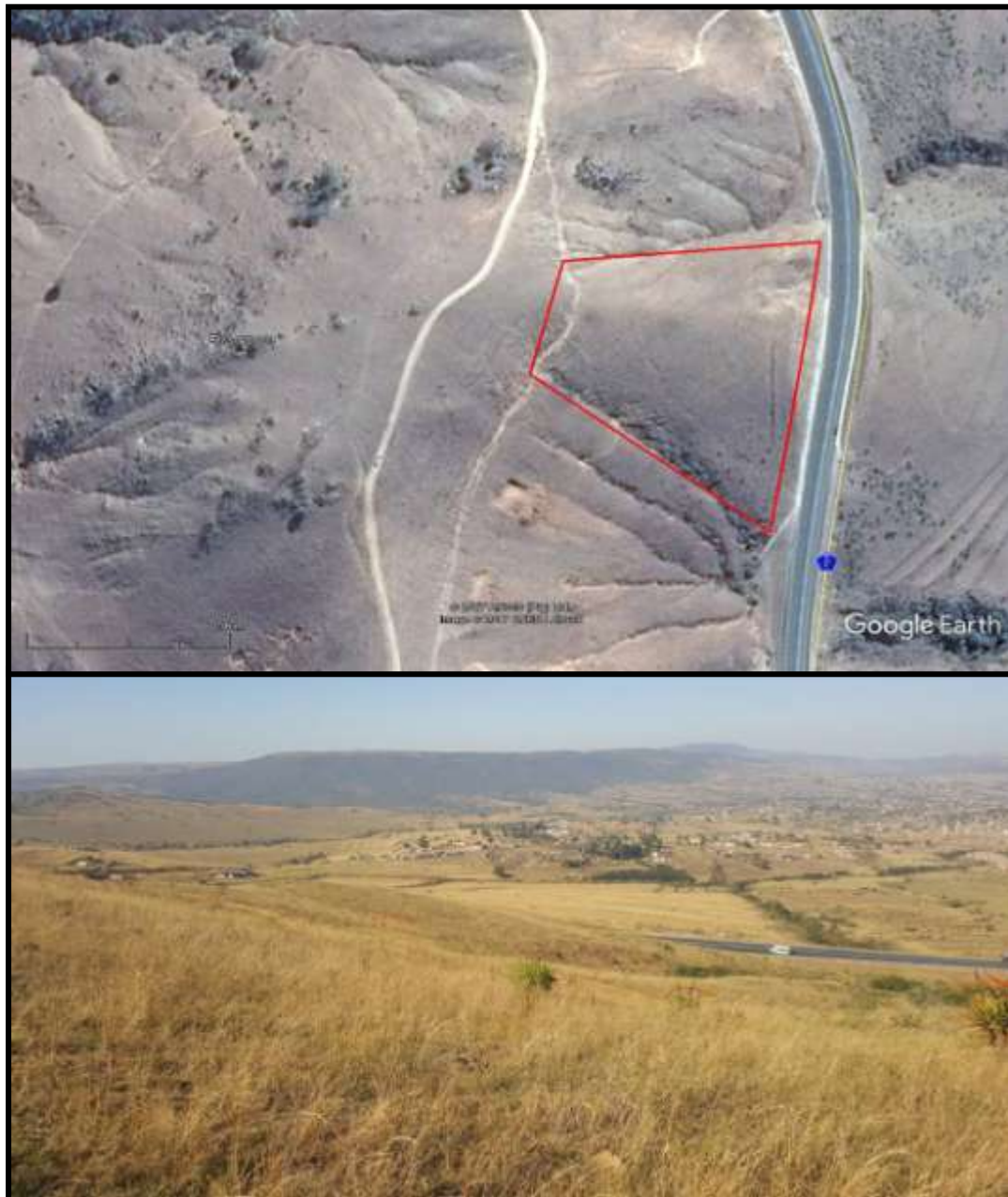
FIG. 10: BORROW PIT 60KM
