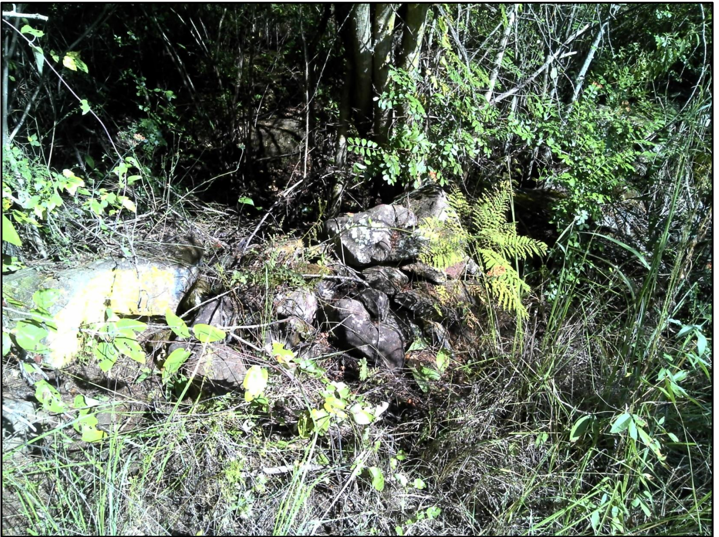
Figure 20: Overgrown stone walling at site 1.
