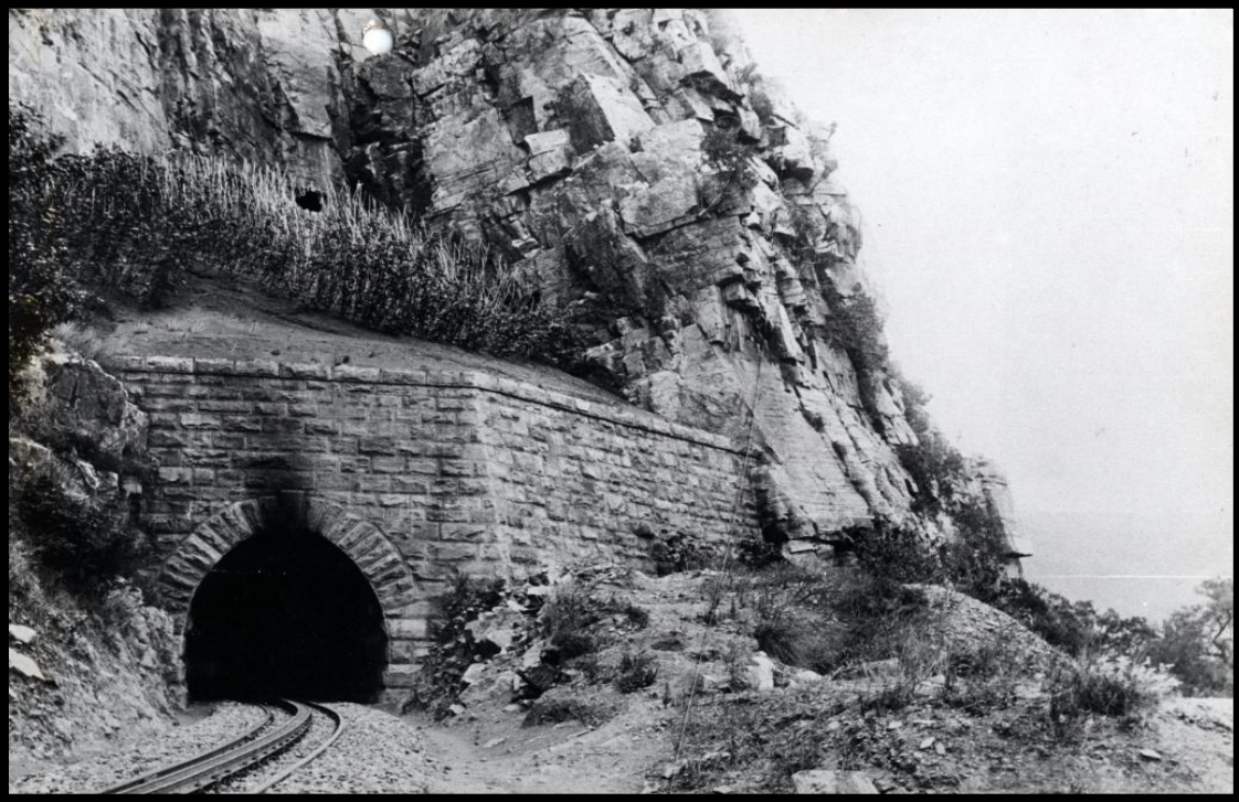
Figure 7: The western entrance of the tunnel. Note the rack-rail in between the normal railway tracks. (NASA)
