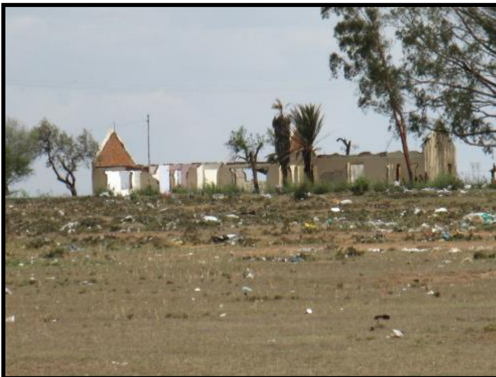
Figure 10. Demolished farm stead (Ruin 4) between the N6 and R702. S 29° 13; 42.72" E 26° 14' 18.16"
