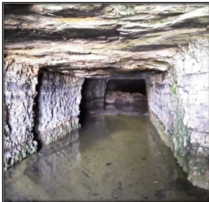
Figure 27: Example of old shaft openings present on the development footprint GPS coordinates: 25,836389S, 29,990556E
