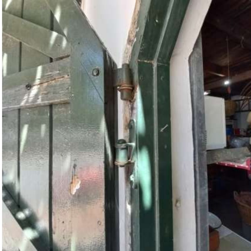
Photo 46. The hinges of the padstal door appear to be relatively recent. Photo: Adolfo Linares.
