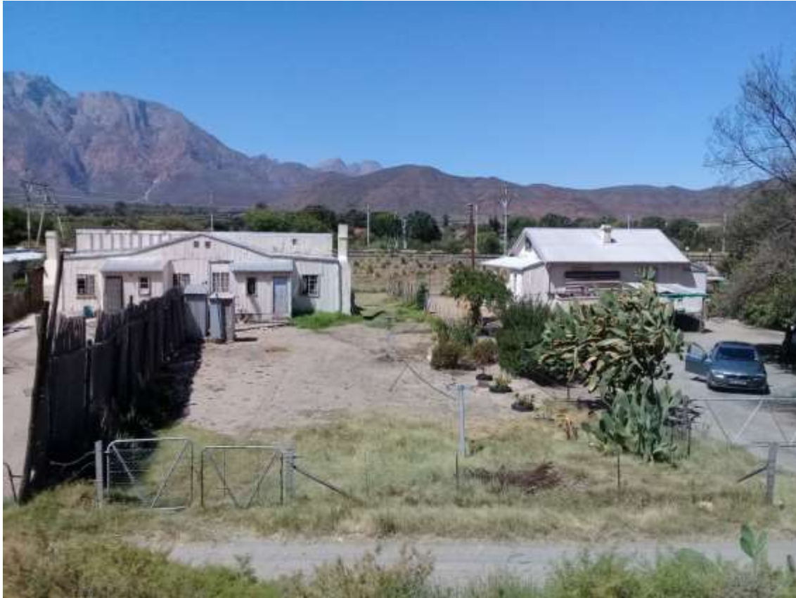
Photo 61. The date of these structures is unknown. A detailed study would be required to ascertain their date and their significance. It is obvious though, that this cluster of houses form a community, and that the proposed freeway (as Options 1 and 2) would be very disruptive, as the residents would lose their houses and would have to be accommodated elsewhere. What they would be paid-out for their houses may not be sufficient for them to purchase something as well-suited to their individual requirements. In addition, their community networks of mutual dependence may also be impacted. It could be that extended families live in these houses. Photo: Sian Hall.
