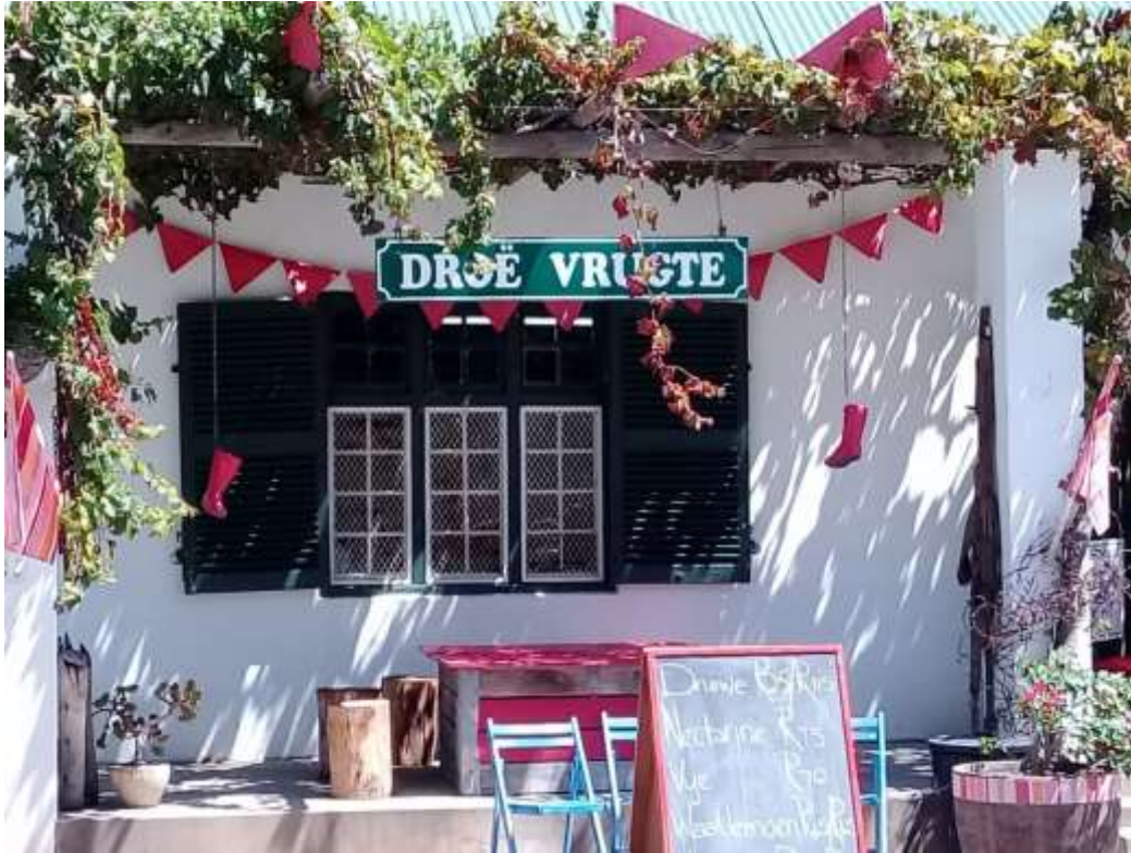
Photo 47. The windows of the building are original. They date to the mid-1800's, or before. Photo: Adolfo Linares.
