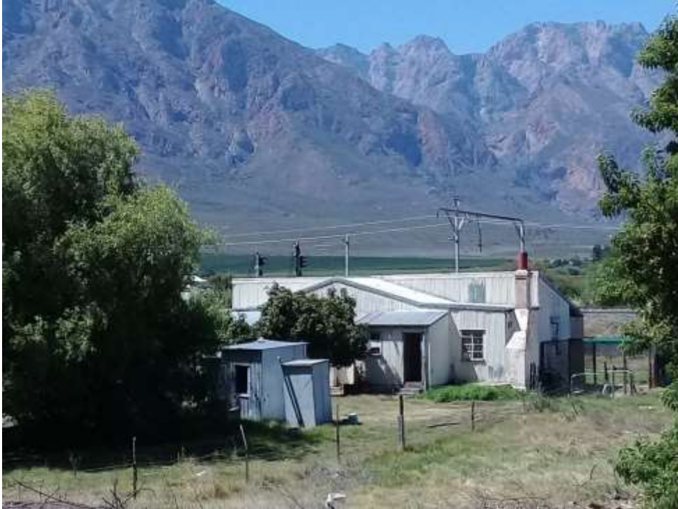
Photo 56. These buildings are built from corrugated Iron sheeting. The length of the sheets, from a distance, appears to be long, but this can only be confirmed on a closer inspection, during a more detailed Built Heritage study. It is quite possible that the material has been reused from an older structure, to build this one. The dates of the buildings are unknown, and can only be discovered during a more detailed study. Photo: Sian Hall.
