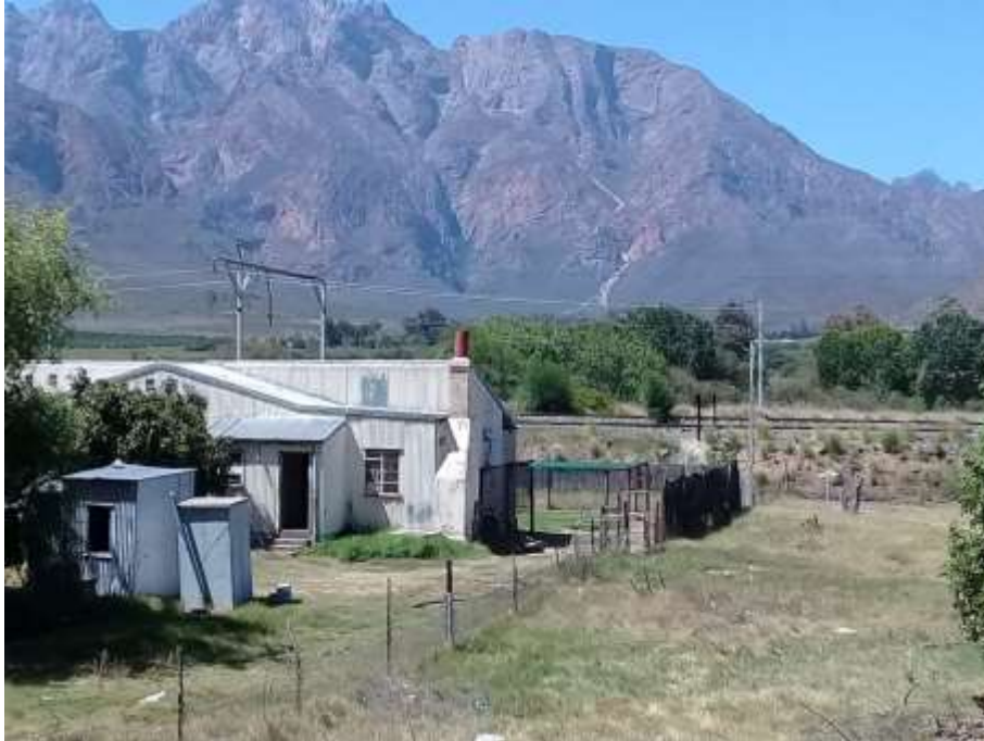
Photo 57. The structures in the foreground are only 7 meters from the N1 freeway. They are built from corrugated sheeting. The structures would be obliterated by the proposed development. The steel windows of the building appear to be a later feature, having been available in South Africa during the 1970's. This photo, taken a little further to the south of the property show, in the background, the valleys and wide open avenues along which colluvium could move down with high velocity water. Photo: Sian Hall.
