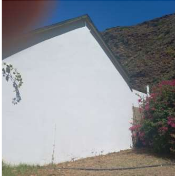
Photo 52. The north wall of the building. Photo: Adolfo Linares.
