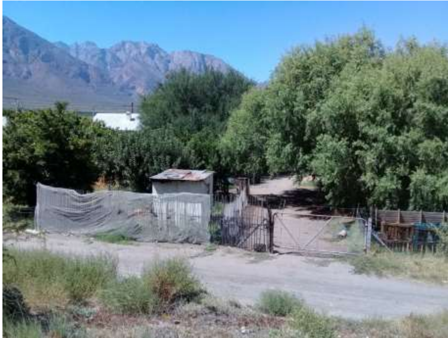
Photo 58. A closer look at the structure that lays closest to the verge of the N1, at a distance of about 7 meters. Photos: Sian Hall.
