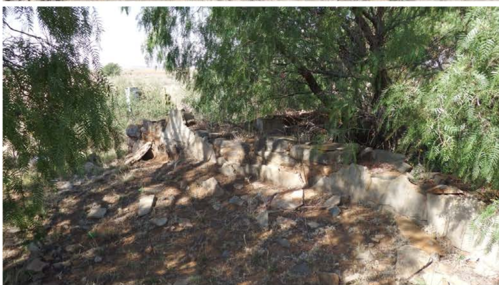
Figure 15. The Brabant pump station (top) and remnants of an old farmhouse located 125 m away to the southeast (center & bottom).
