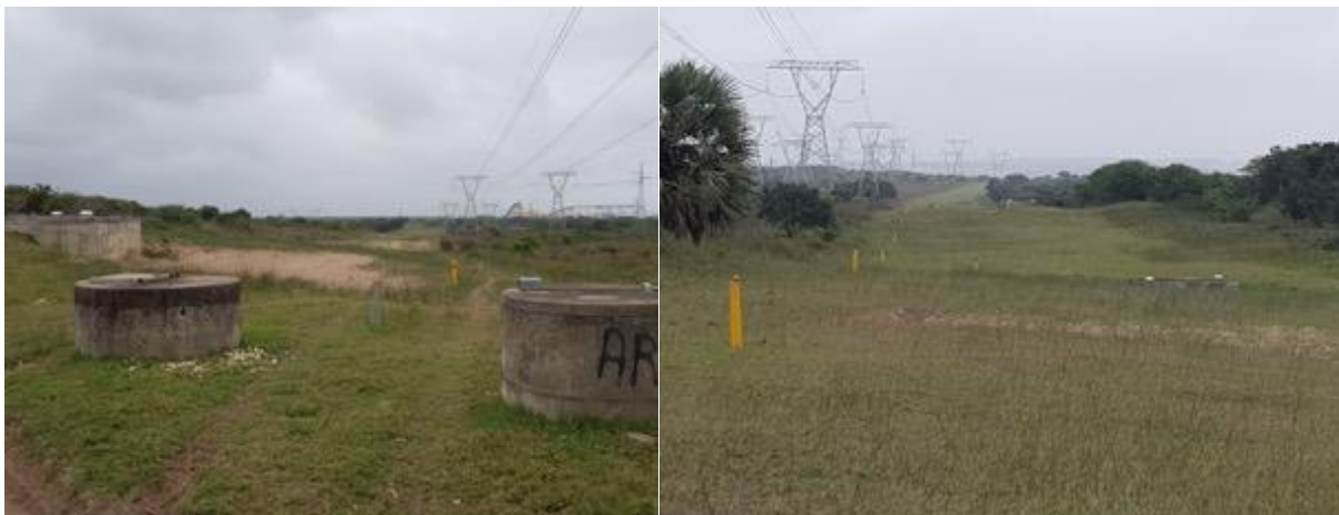
Figure 13: Water infrastructure and servitude along the existing Powerlines and west of the TransNet railway line
