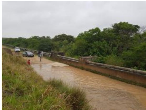
Figure 9: Sewer and water pipelines
