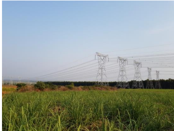
Figure 7: Example of existing Powerlines in East-West Study Area
