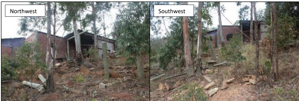
Figure 21: Northwest and southwest corners of the main house.
