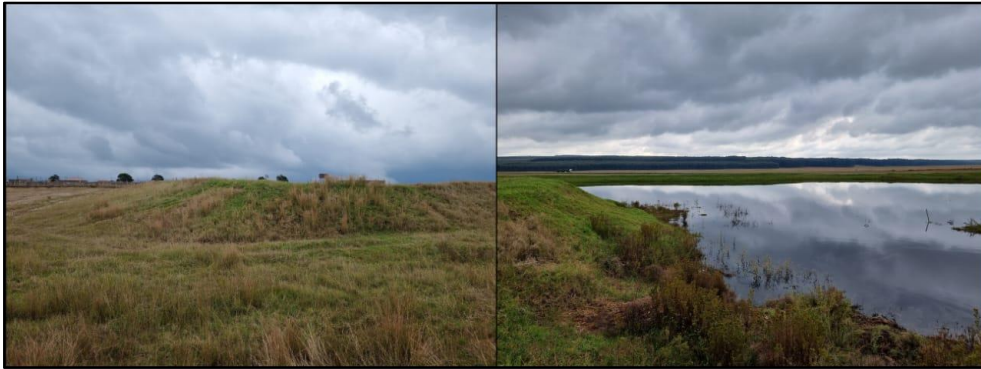
Figure 4-6: View of the old slimes dams in the project area.
