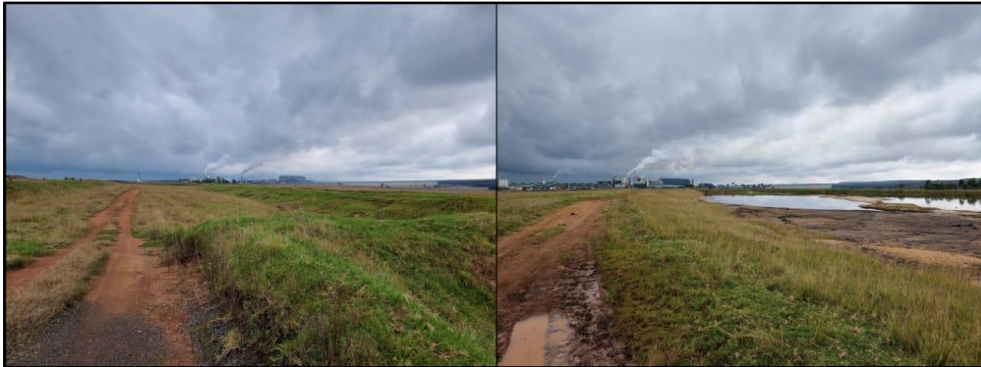
Figure 4-7: View of old cascading dams in the project area.
