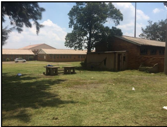
Figure 6: General Site conditions
