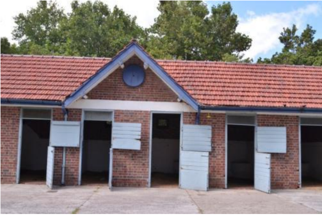
ABOVE: EXISTING STABLES.
