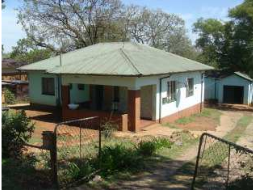
Figure 8: Another type of old house in Salvokop.
