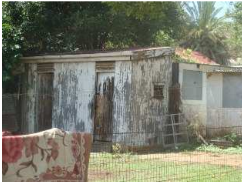
Figure 15: A corrugated iron building at one of the houses.
