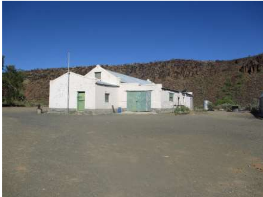
Example of built heritage (site BHS-5)
