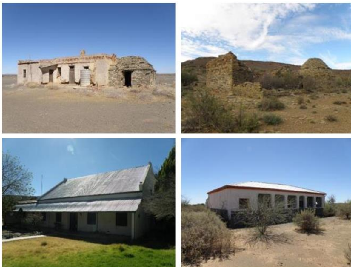
Figure 6-6: Examples of Corbelled Houses (Top) and Late 19 th , Early 20 th Century Farmstead Houses (Bottom) Assessed during the In-Field Survey
