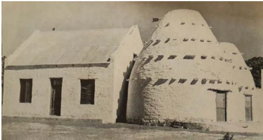
Figure 9: Stuurmansfontein homestead with two linked corbelled rooms with a later pitch roofed rectangular room and a flat roofed rectangular building (VASA 2007:55)
