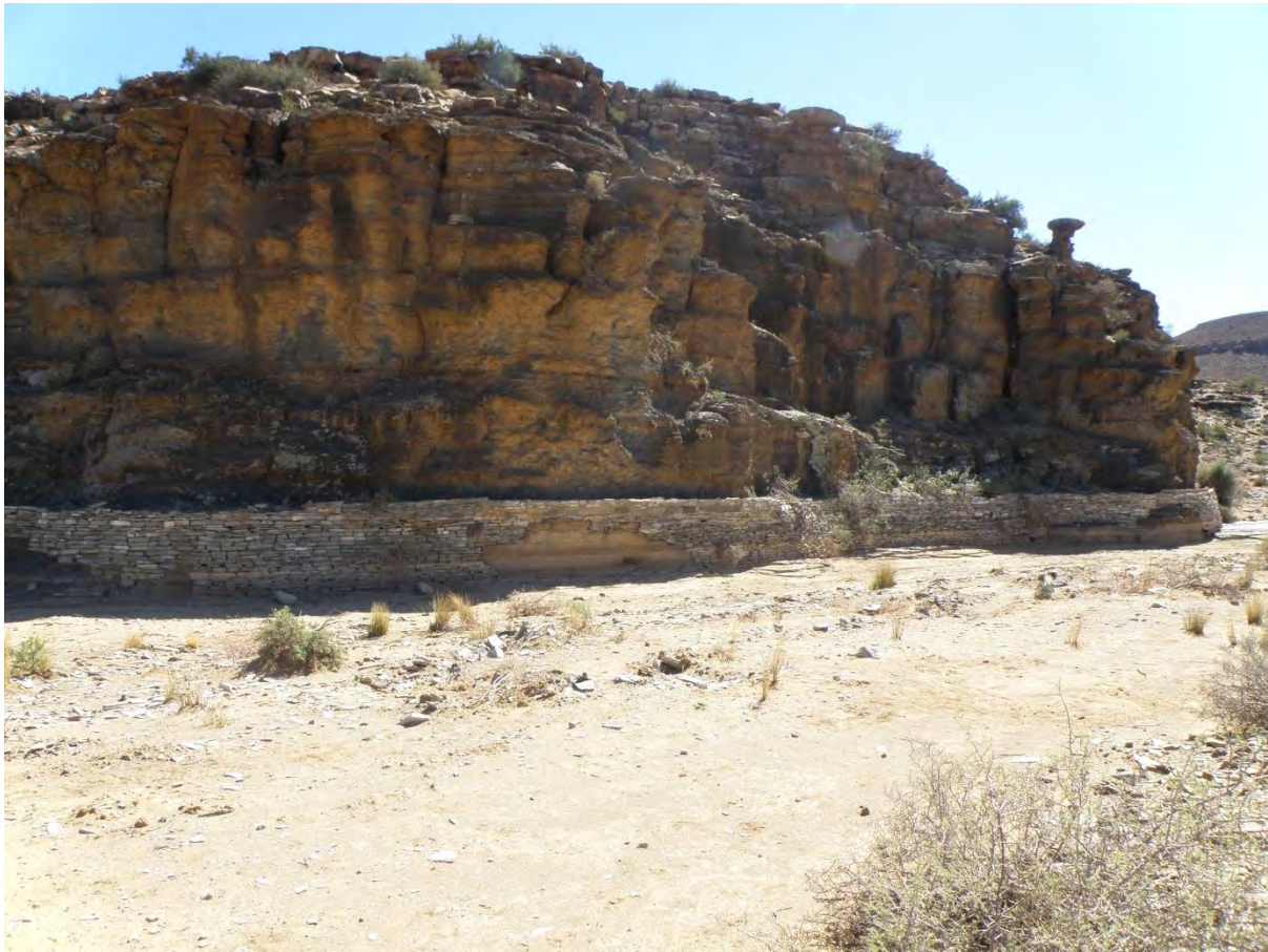
Figure 18: Retaining walls along bas of cliff
