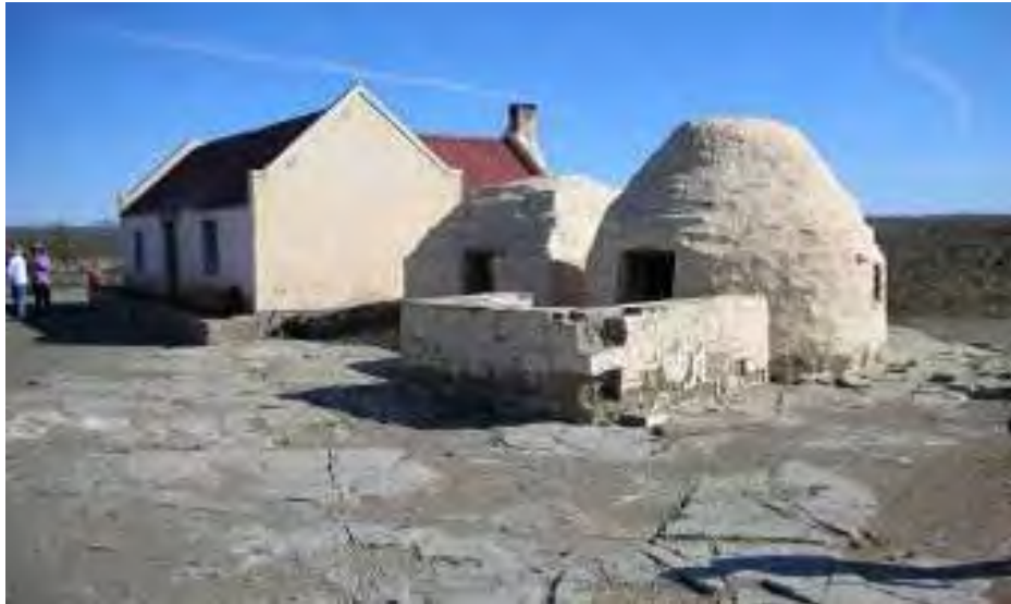
Figure 8: Vischgat homestead showing the evolution of architectural styles including circular corbelled hut, square corbelled hut and T plan pitch roof house with a brak dak buite kamer attached (VASA 2007:58)
