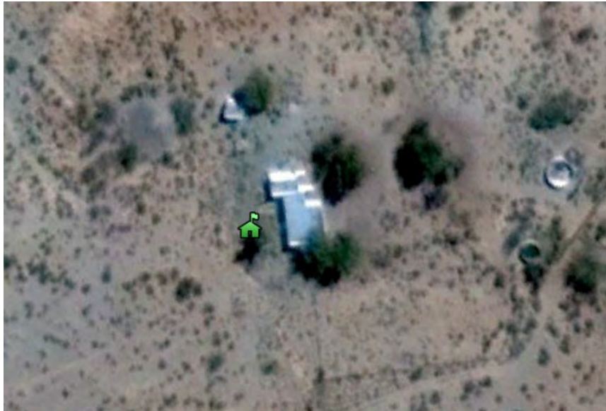
Figure 15: Aerial view of building
