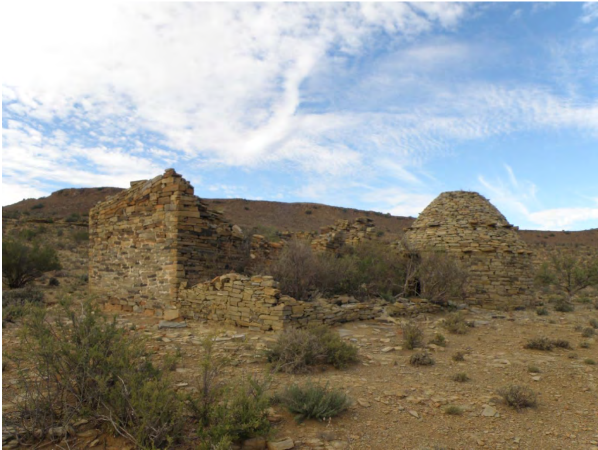
Figure 17: Corbelled house with collapsed later addition
