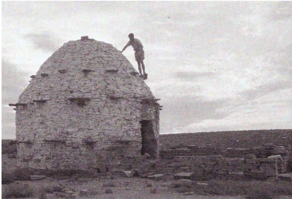
Figure 6: Gawie Fagan illustrating the speculated use of projecting stones as scaffolding for construction and roof repair (Fagan 2008:38)
