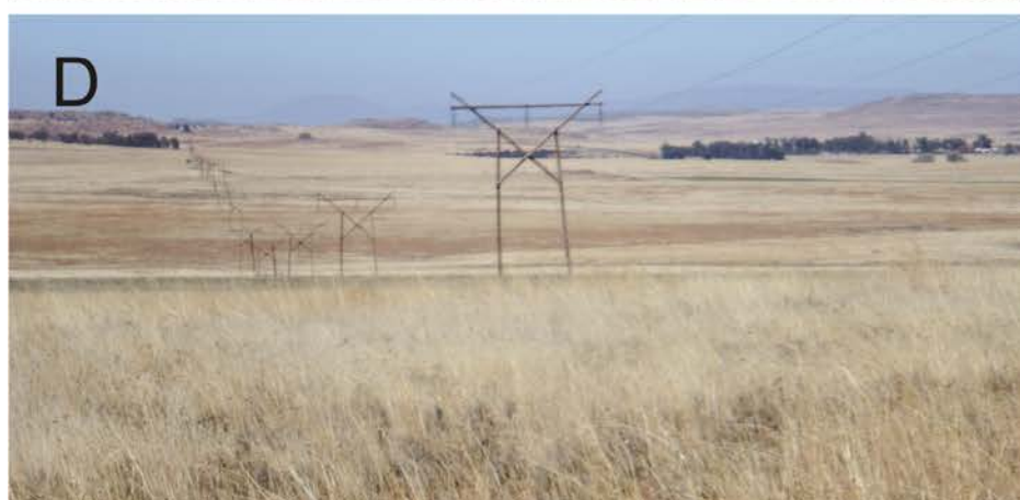
Figure 3. General view of the Rouxville Substation and footprint between route section A-B.
