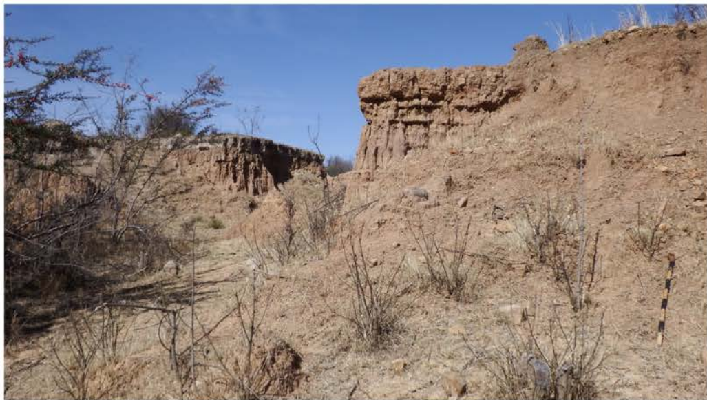
Figure 11. Pipeline section running south of the mountain and east in the direction of Ficksburg (top). This section is characterized by extensive erosional gullies (dongas) flanking the spruit.
