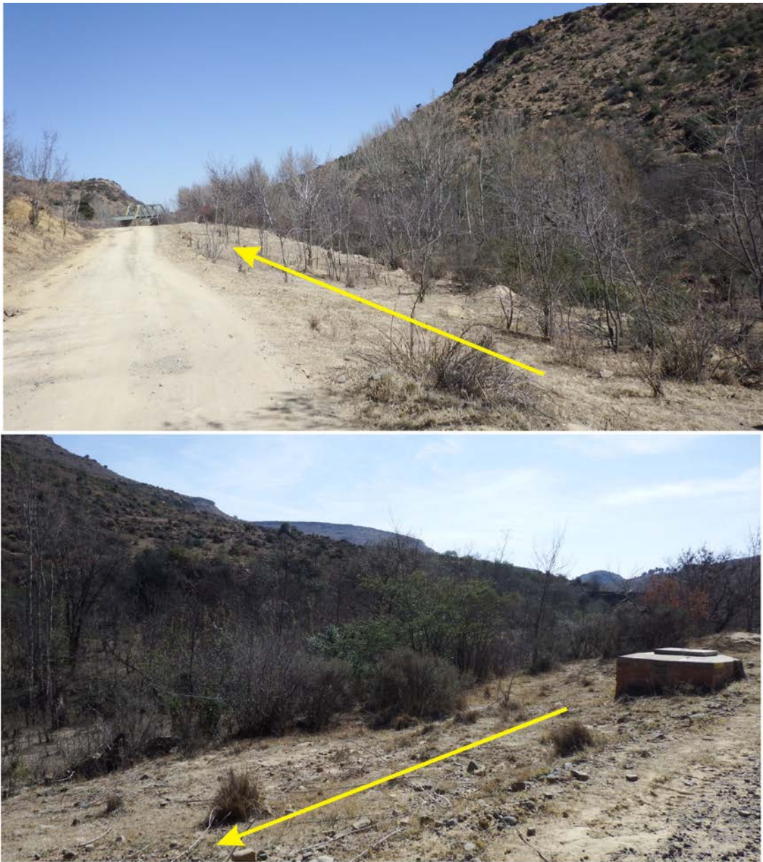
Figure 7. Pipeline section south of the Meulspruit Dam flanking the spruit, looking southeast (top) and northwest (bottom).
