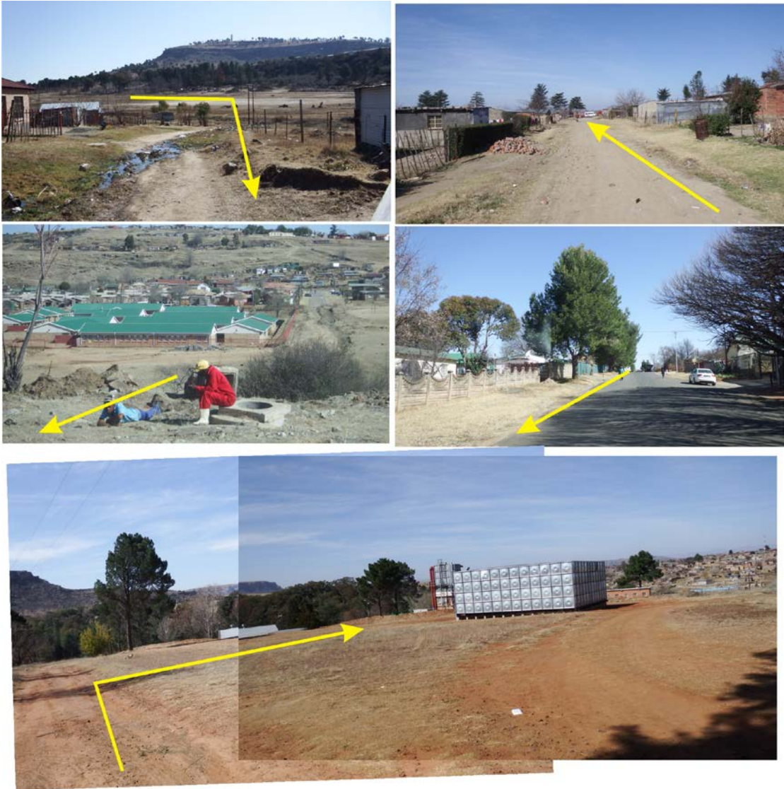
Figure 13. The pipeline footprint traversing residential areas in Ficksburg, terminating at the water treatment works at the Caledon River (bottom).
